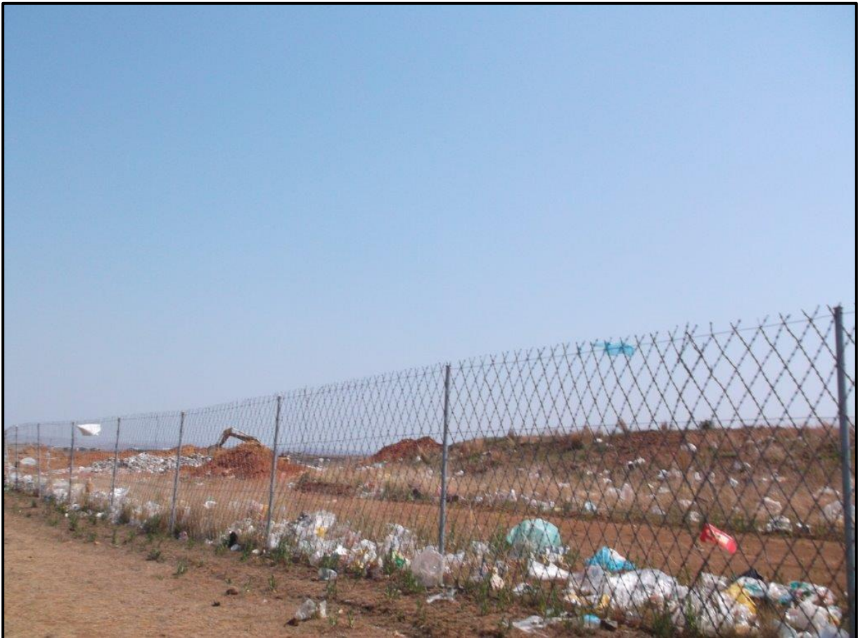
Figure 7: Unlined Landfill Site; No Berms or Trenches Present
