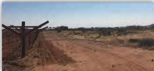
Figure 11: Scarifying of soil
