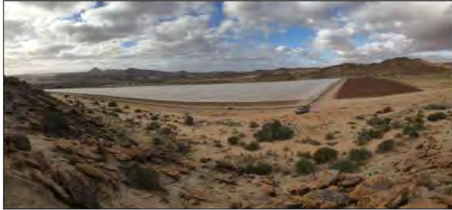
Figure 8. Block 3 (22ha). View facing north east
