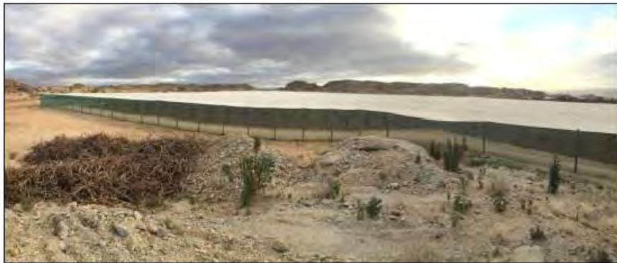
Figure 6. Block 1. View facing north west
