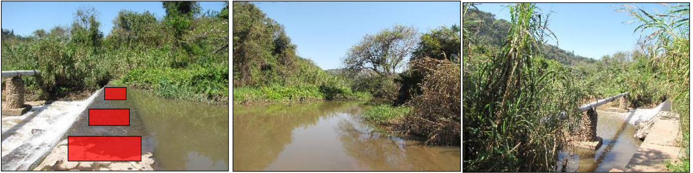
Figure 7: Photographs of the existing weir across the Mhlatuzana River
