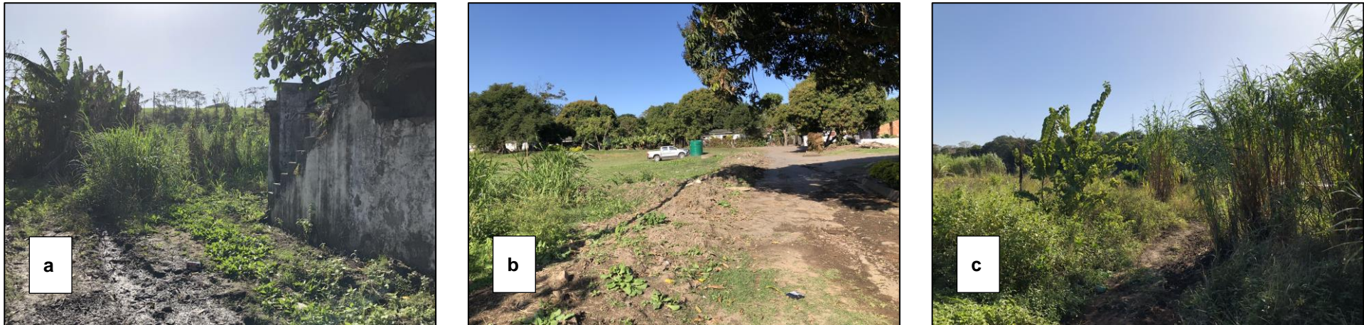
Figure 2: (a) View of the current pump dilapidated station; (b) View of the public open space where the rising main will be located; (c) View of the overgrown disturbed site looking south west.
