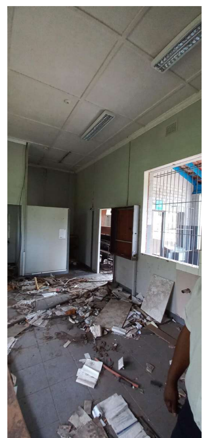
1. EXISTING STATION BUILDING - INTERNAL
