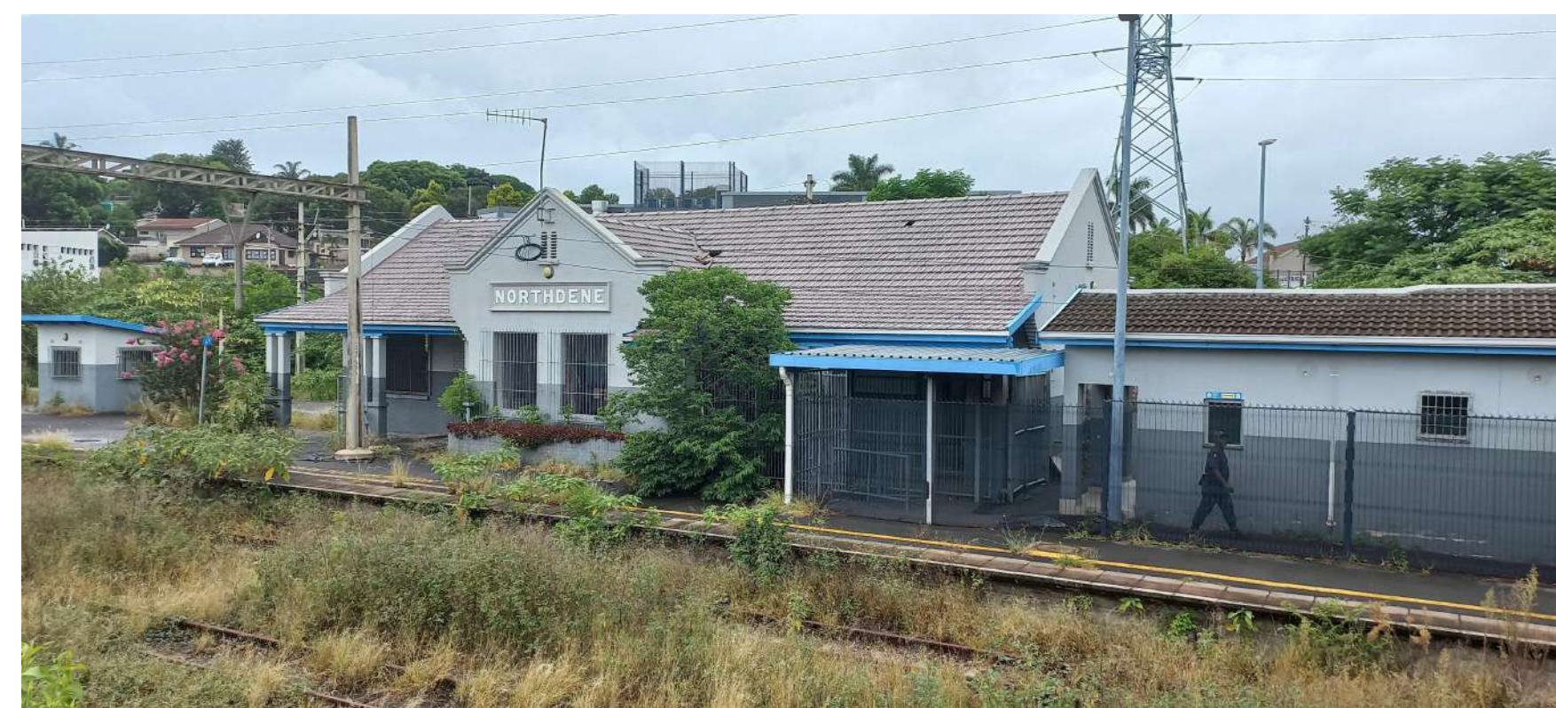
5. EXISTING STATION BUILDING
