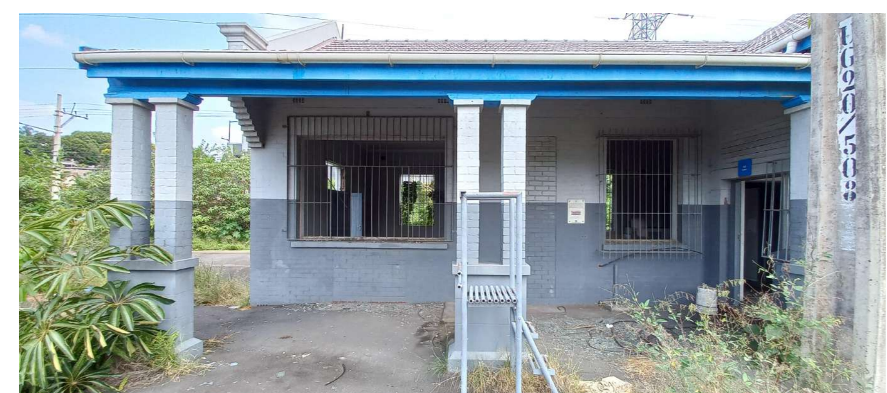
6. EXISTING STATION BUILDING
