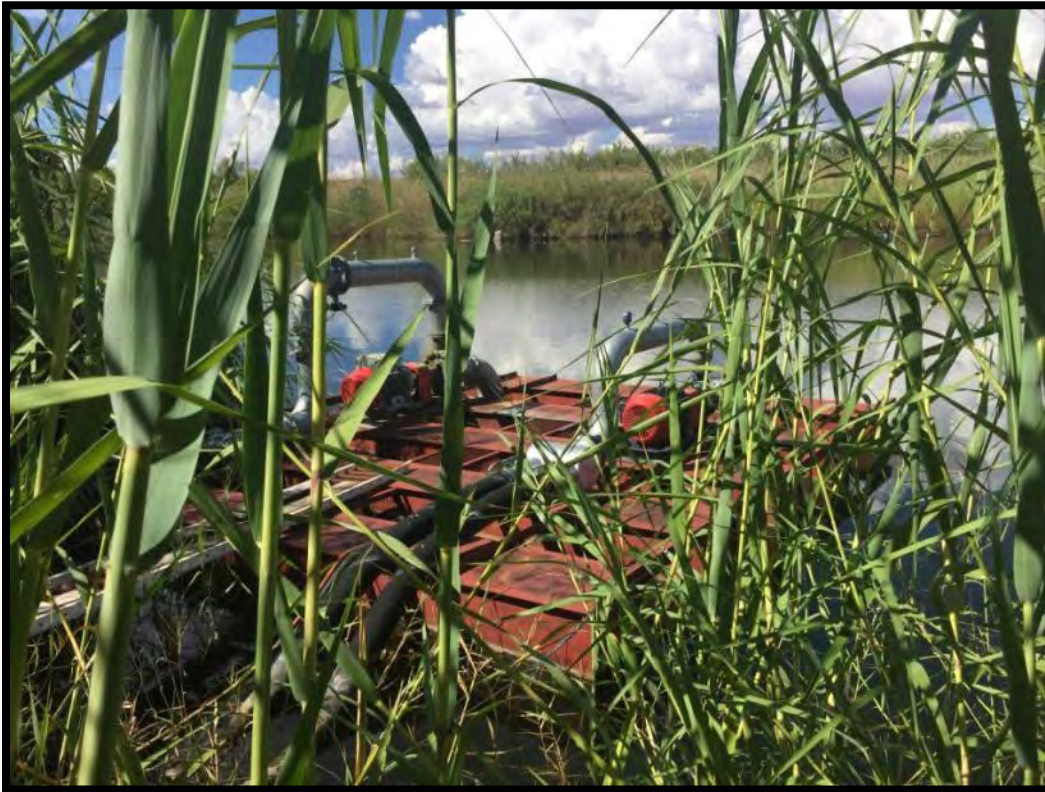
Pump – Intake off the Orange River
