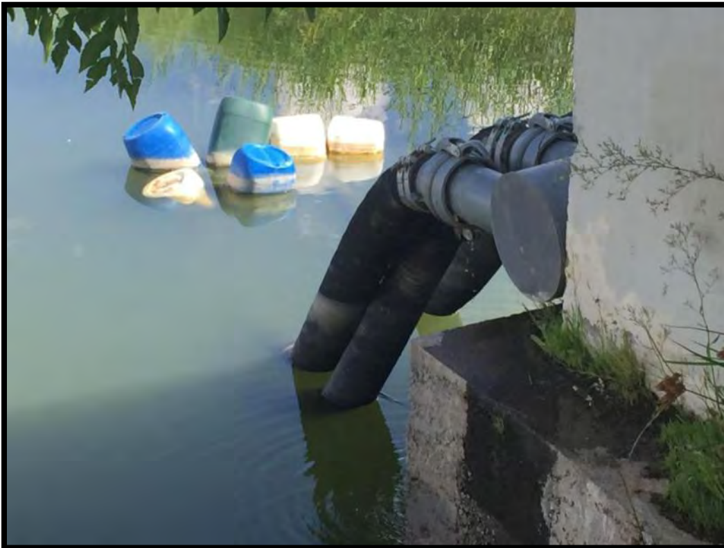
Pump – Intake off the Orange River
