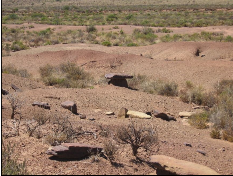
Figure 12. Highly eroded ground in the north-western part of the site
