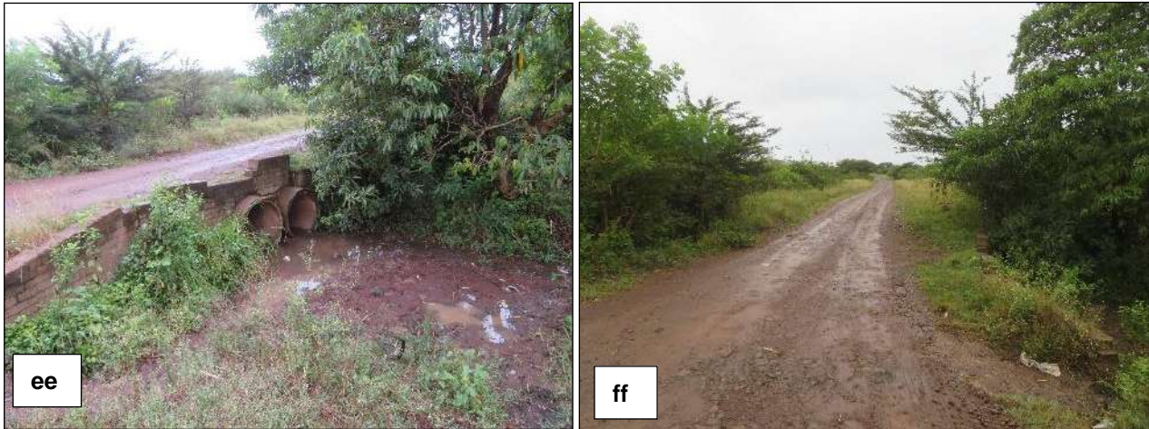
(ee) View of two pipe culverts crossing Manzakata river downstream of WC21; (ff) The road servitude and dense vegetation associated with WC21.
