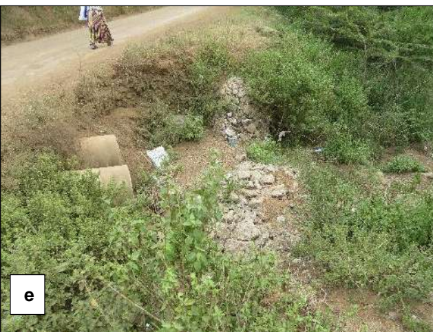
(e) The rocky crossing in the channel at WC4. There is a 2 pipe culvert in place for the road crossing in this watercourse.; (f) View of a bridge crossing over Jenga River at WC5.
