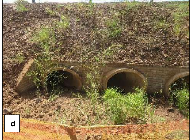
(c) View of a wetland adjacent to WC2.; (d) View of three pipe culvert crossing at WC2.
