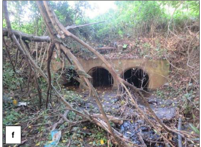
(e) The dense vegetation and wetland associated with WC3; (f) An existing concrete 3 pipe culvert is present at WC3.
