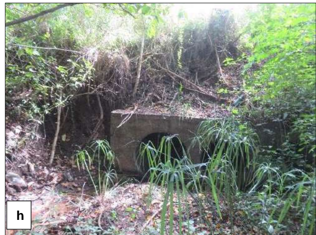
(g) Overview of indigenous vegetation at WC4; (h) The existing concrete pipe culvert associated with WC4.
