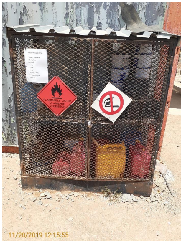
Photo Plate 8. Hazardous substances stored in a designated ventilated storage area with spill containment.
