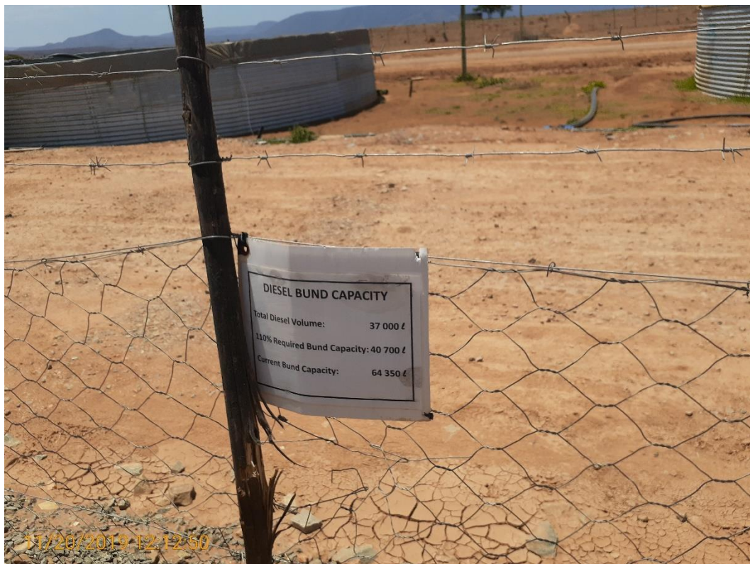
Photo Plate 4. Indication of the tank and the bund capacity at the Diesel storage area.
