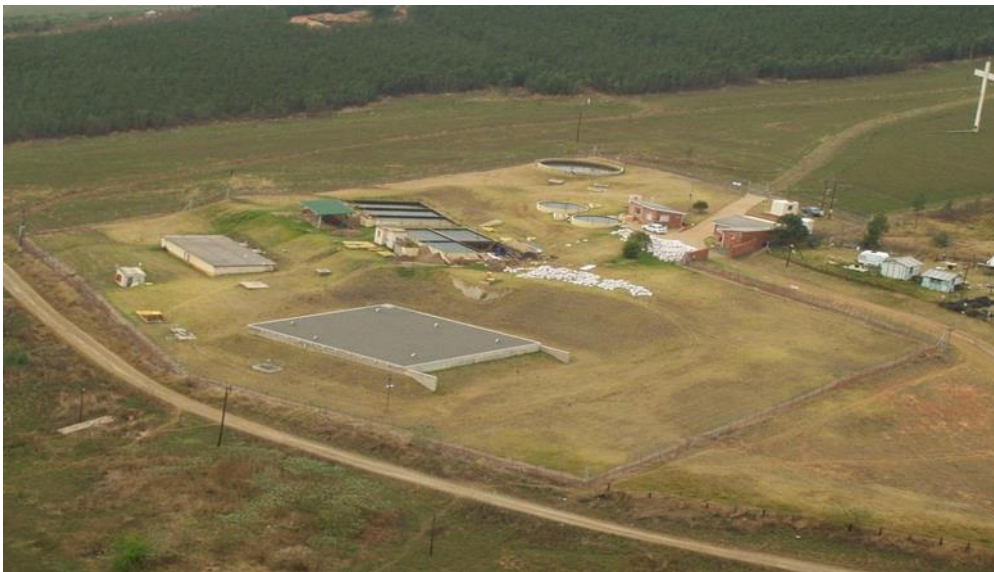
Figure 4-Ixopo Water Treatment Plant (Umgeni Water Amanzi - Planning Services, 2022)
