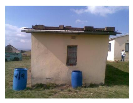
This is the right side elevation. Once again the back wall leaning outwards is clear. The façade shows signs of being touched up recently, so there are no obvious cracks, but we expect them to appear due to the leaning wall. Note also the condition of the roof. The sheets will need to be replaced.
