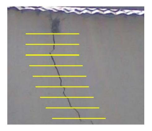
The photograph above shows typically how "stitching" will be carried out, using one metre long lengths of 10mm diameter high yield steel reinforcing bars.
