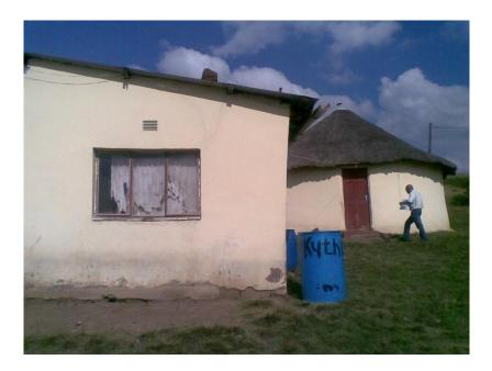
This photograph shows the right hand side of the front elevation. The right side wall is leaning outwards such that it has caused a tension crack in the front wall.
