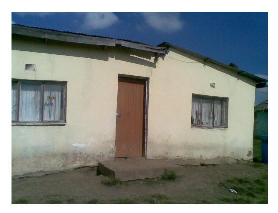
This view, the front elevation, clearly shows that the roof timber has rotted. The window and door frames are in poor condition. The walls have cracks above the windows and door. There are also indications of rising damp. The top part of the wall on the right hand side is leaning to the right. The walls are of concrete blocks as can be seen in the exposed portions.
