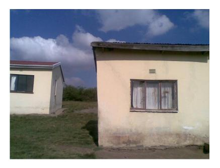
This photograph shows the left hand side of the front elevation. The wall on the left is leaning towards the left and has resulted in the formation of the crack in the front wall.
