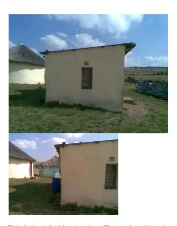
This is the left side elevation. The back wall leaning outwards can be clearly seen.
