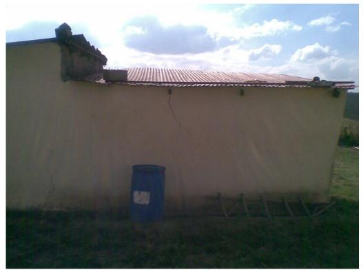
The two photographs above show the whole back wall. The left and right walls are leaning outwards in each case. The back wall itself has two full height cracks, from the ground to the roofline. One is by the change in height of the wall, which is reflected at the front wall above the doorway and the other is just right of the blue drum.
