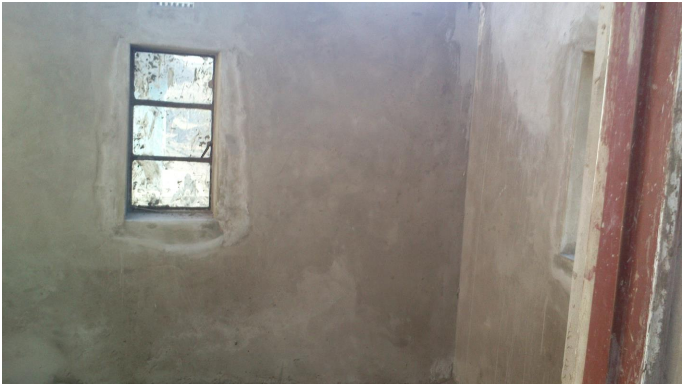
Image 006 Indicating Internal new plaster work on walls
