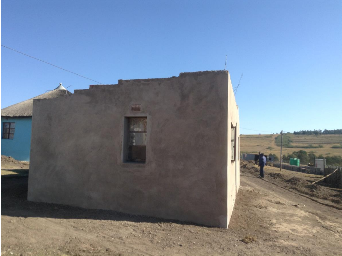
Image 008 Indicating Internal new plaster work external walls
