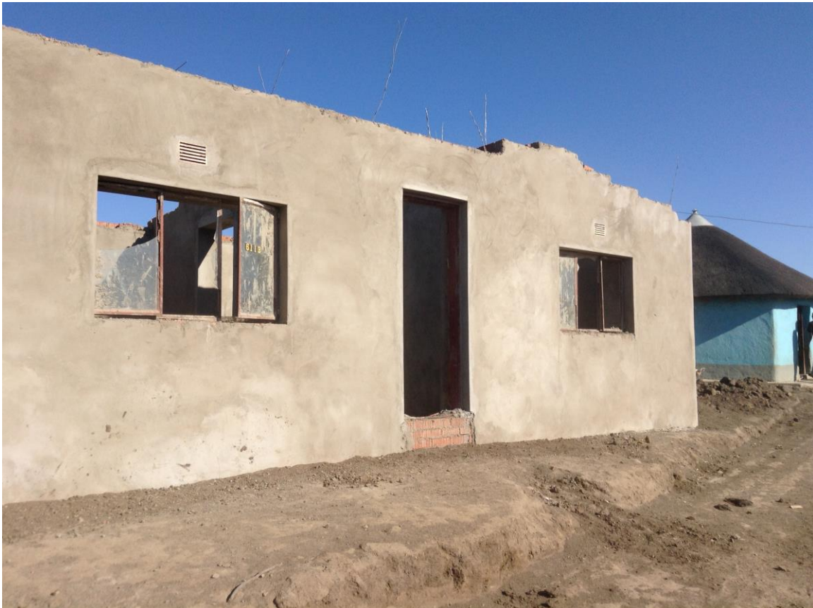
Image 009 Indicating unaffected window, doors and ventilation openings on external walls
