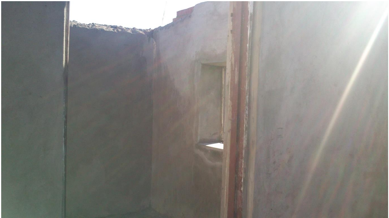
Image 007 Indicating door frame and in background window opening and internal cill
