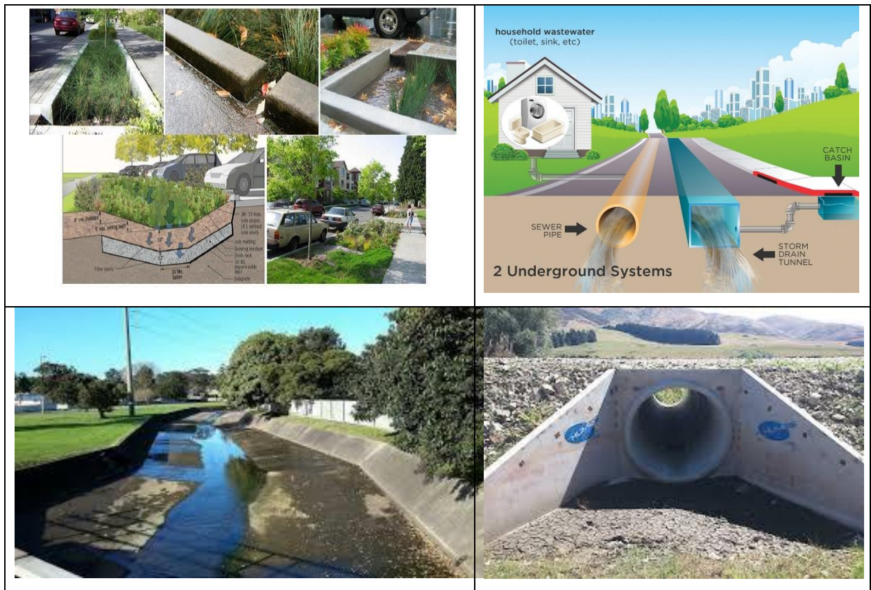
Figure 3- Typical Well Maintained Stormwater infrastructure
