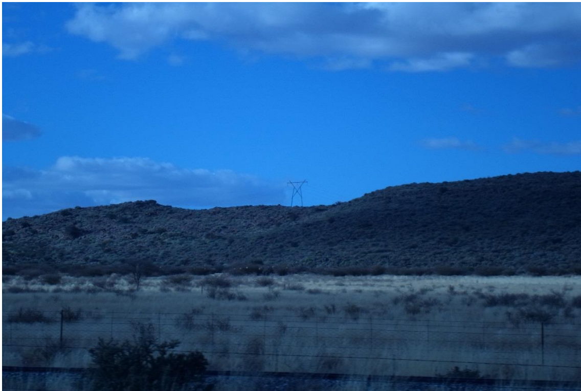
Figure 9: View of the Oasis-Taaipit 132Kv Powerline coming over the ridge.
