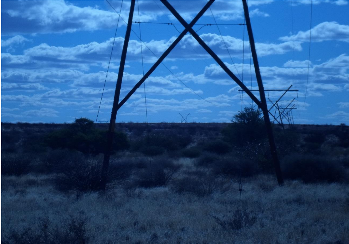
Figure 6: View along the Oasis-Taipit 132Kv Powerline
