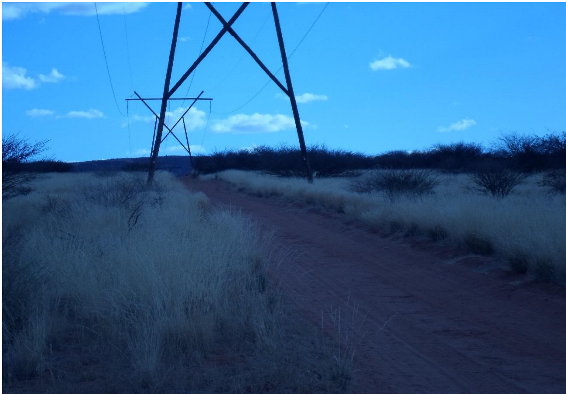
Figure 7: An access road running under the Oasis-Taipit 132Kv Powerline
