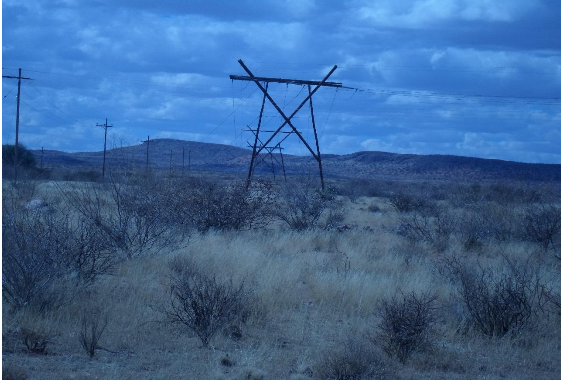
Figure 2: View of the Oasis-Taaipit 132Kv Powerline moving away from the Oasis Substation
