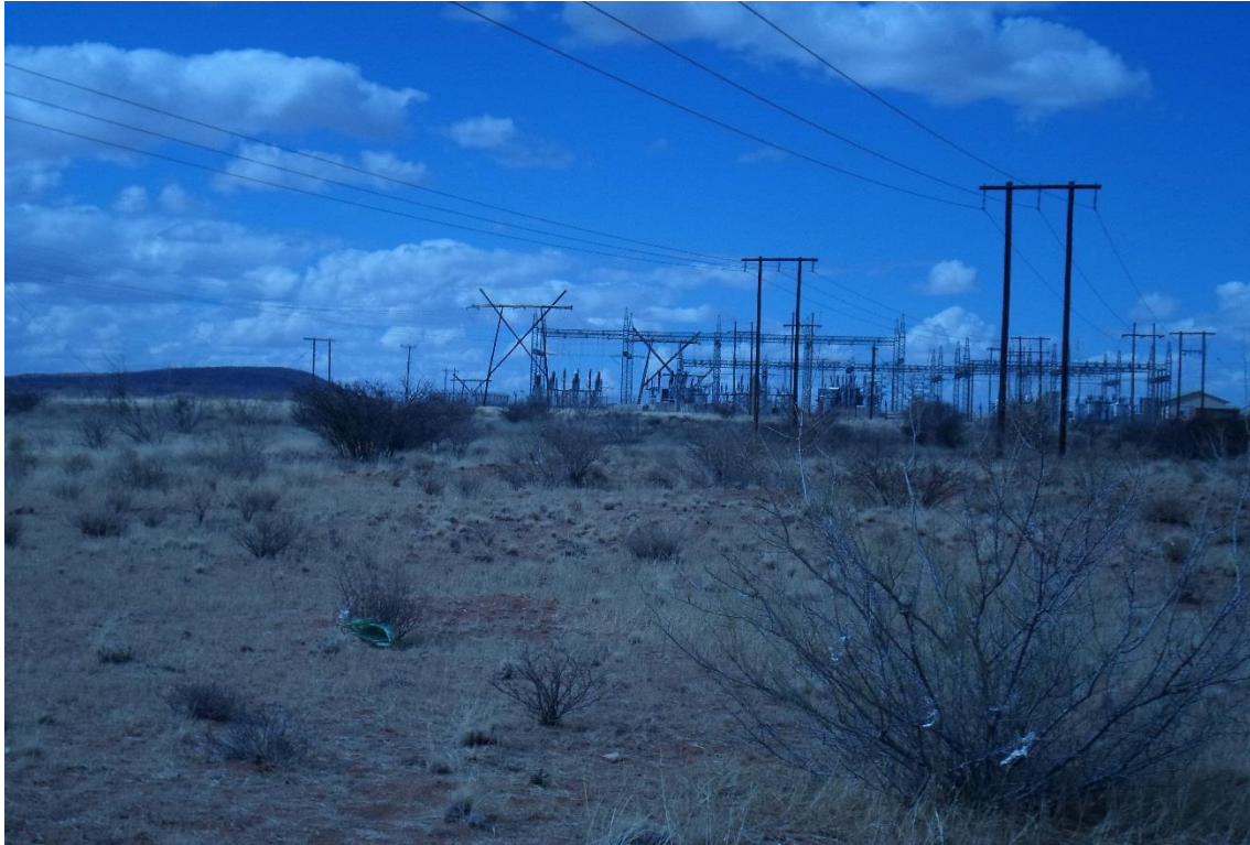
Figure 1: Existing Oasis Substation
