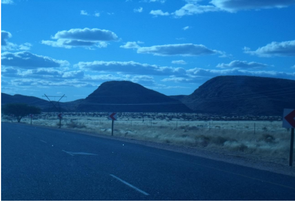
Figure 8: Roadside view of the Powerline running next to the N14 Road.
