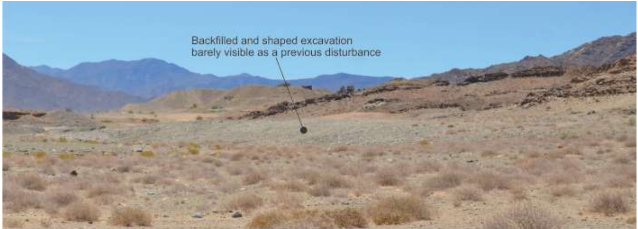
Photo 12: Backfilled and shaped excavation (and dump area) in the west of Oena
