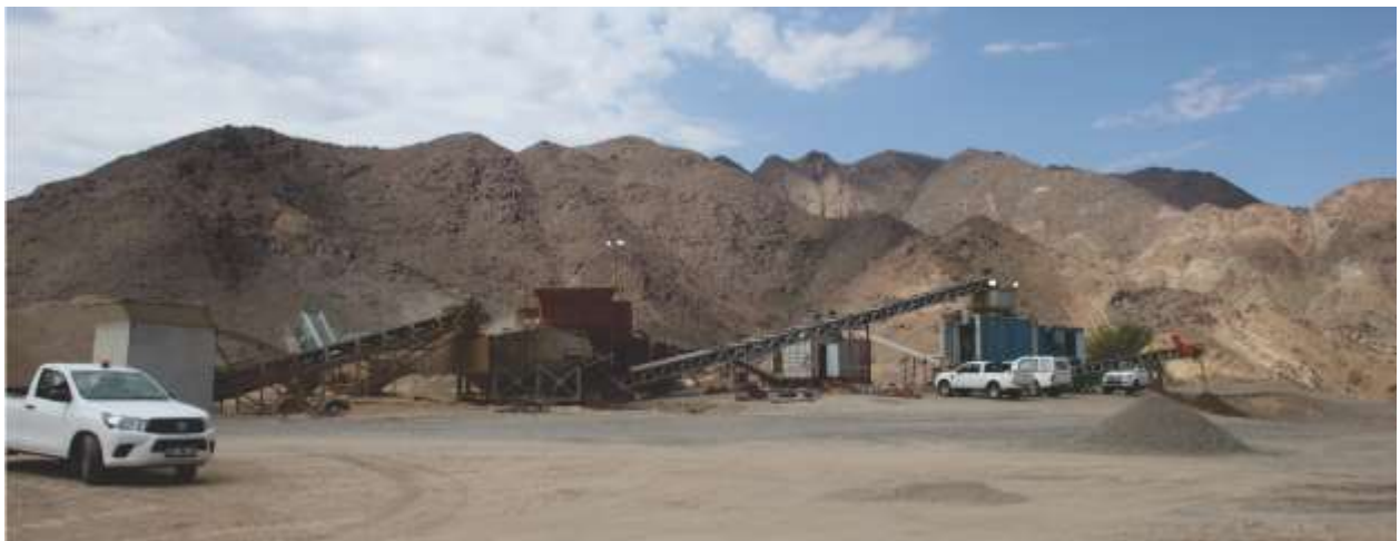
Photo 4: The static plant located on top of the main coarse waste rock stockpile (with recovery plant on the right)
