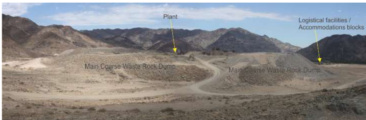
Photo 3: View of the main coarse waste rock dump from the top of the Barker pothole site
