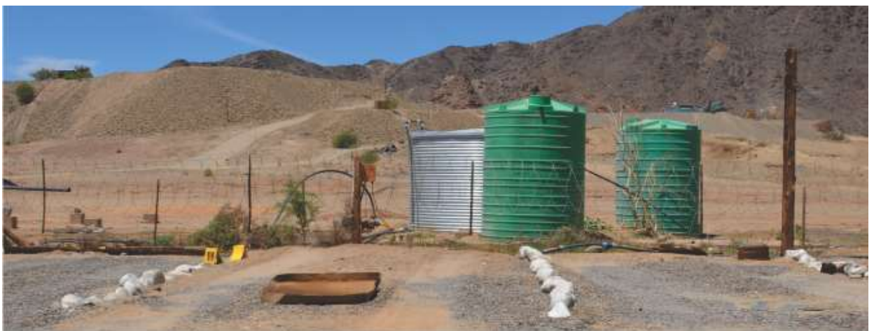
Photo 11: Drip trays in position at the equipment parking bay
