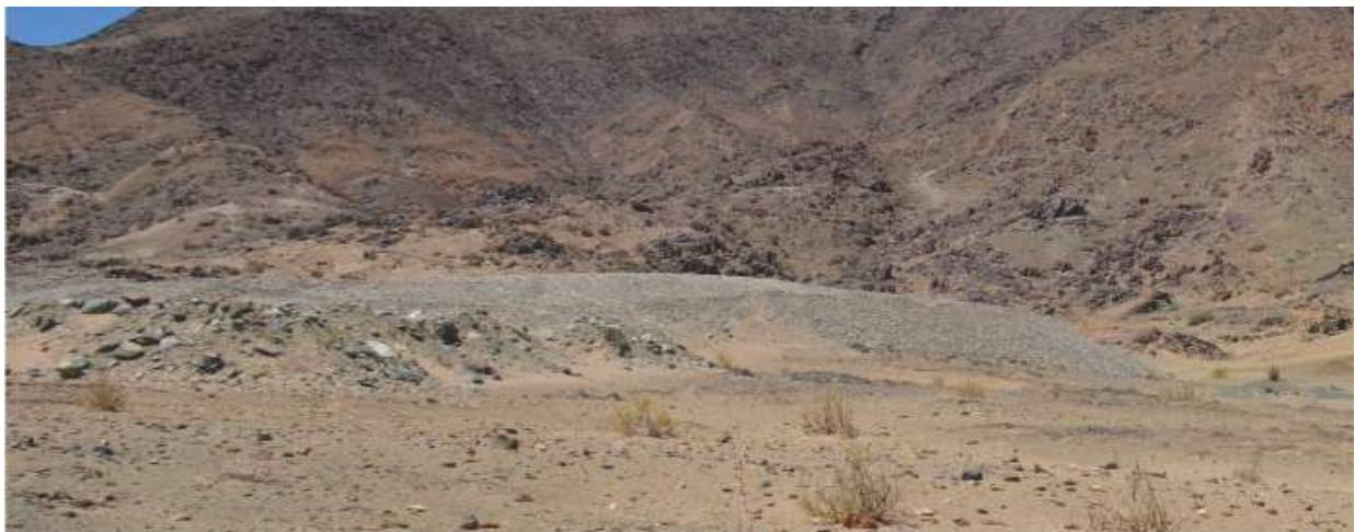
Photo 13: The far western waste rock dump, partially shaped and rehabilitated. The foreground dumps must be levelled or used as backfill for adjacent pits when applicable
