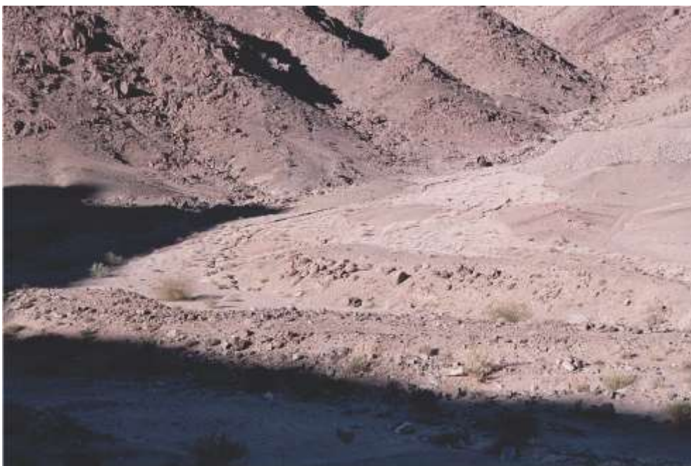
Photo 10: Looking up the valley in the western end of Sandberg where previous processing and in field screening plants were located. Some work as described in the text is required to finally shape the site and rehabilitate old unconfined fine tailings run-off
