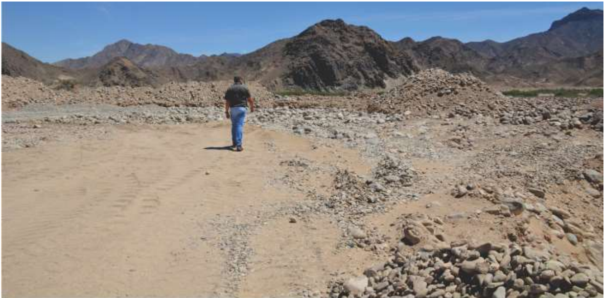
Photo 2: Walking on backfilled excavation in the Oena East Mine block
