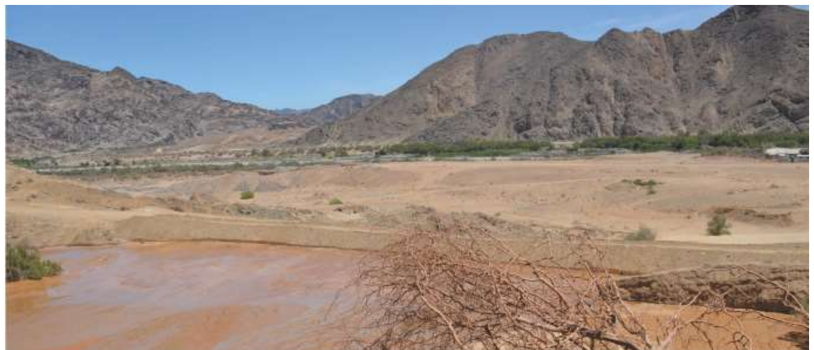
Photo 14: Newly constructed Fine Tailings Dam wall for the Oena Main Plant
