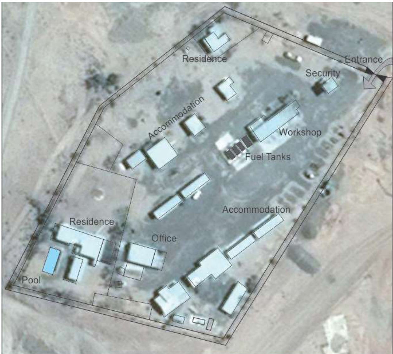
Figure 8: Logistical Facility Area
