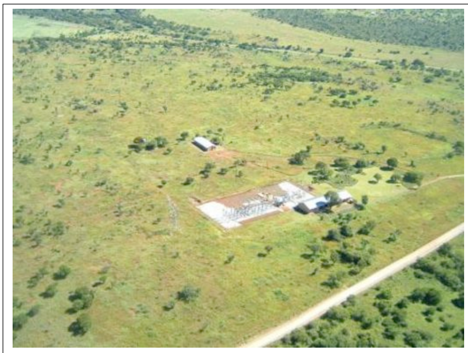
Figure 24- The Ohrigstad Substation to the west of Drakensberg near the historical (older) Ohrigstad in the southern part of the Eskom Project Area (above).
