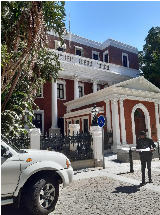
Front façade facing Parliament street (2020) : View of the 2 nd floor before the fire, showing the detailed plastered features.
