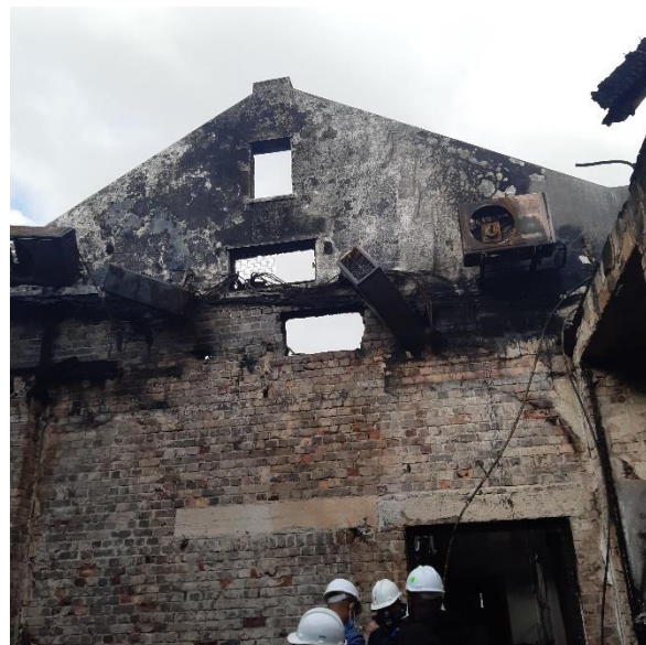
Picture 8 : Close-up of gable wall
