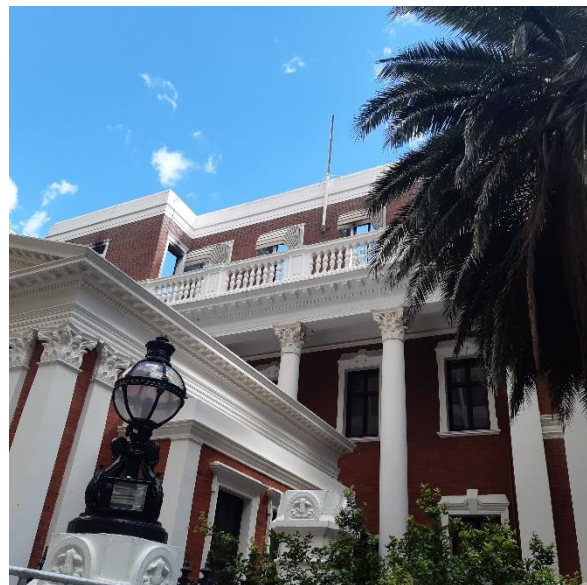
Picture 12 : External view of facade
