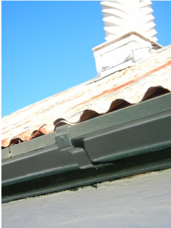
Existing Gutters to be retained
