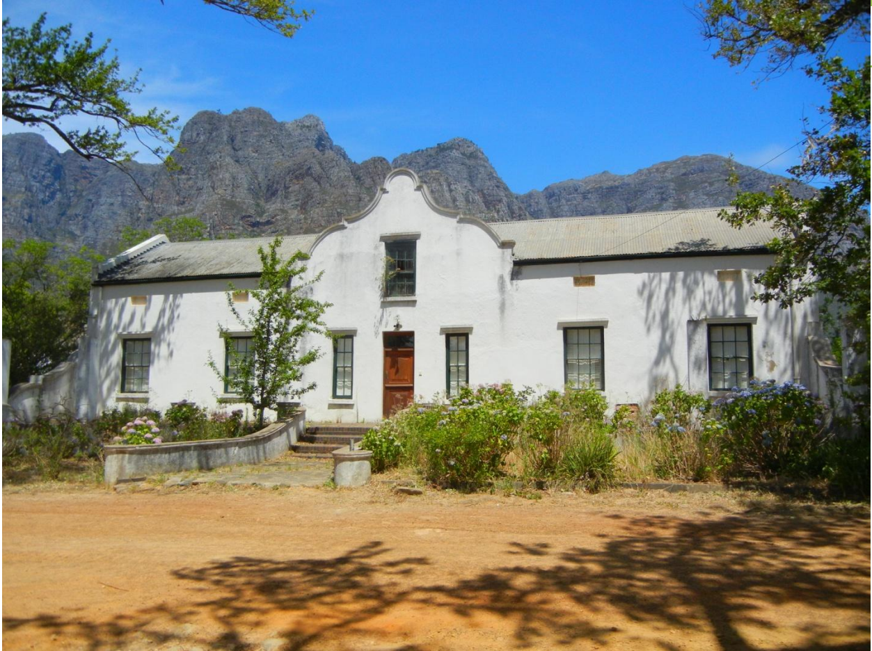
Existing Front Facade
