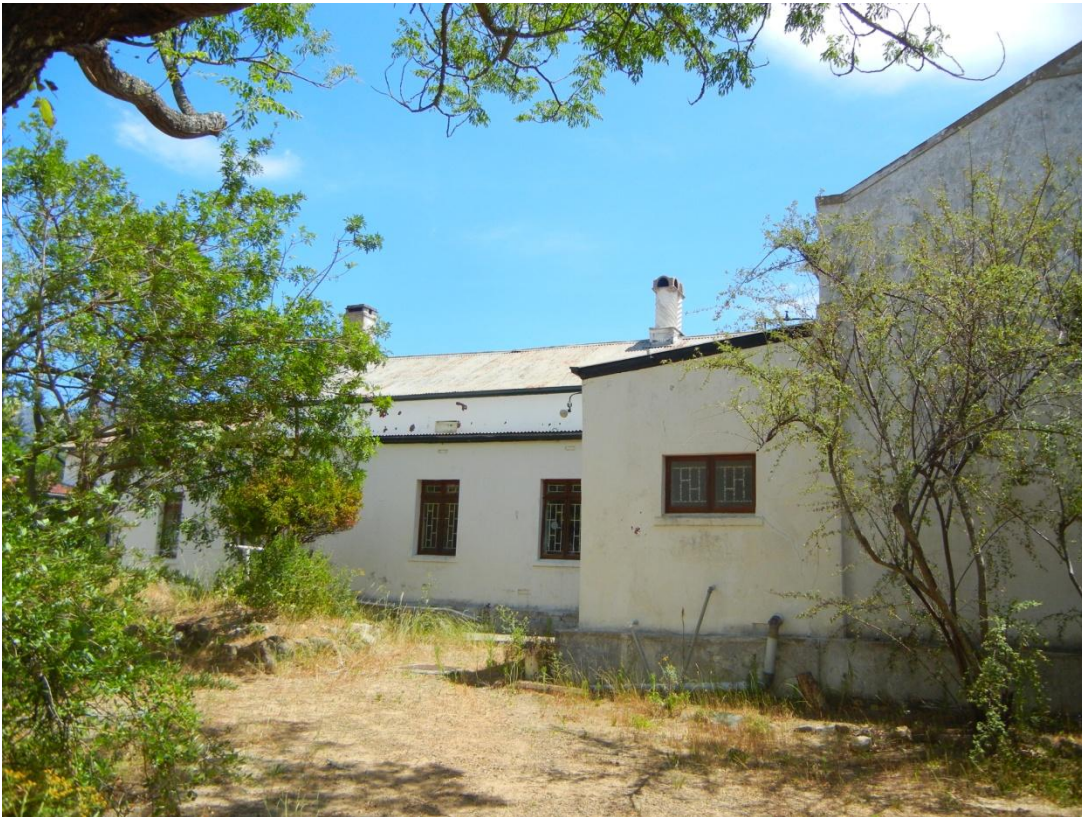
View of Lean To service structure on Kitchen Werf side
