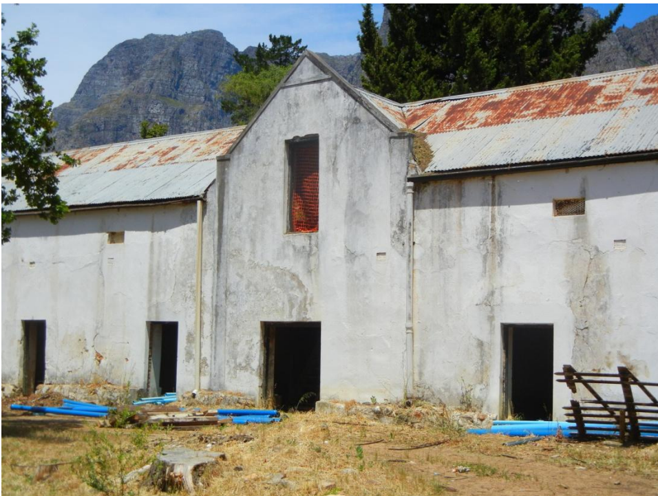
View of Stable Building – Roof sheeting to be replaced
