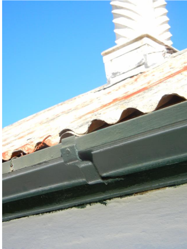
Typical existing Galvanized Gutter & Bracket
