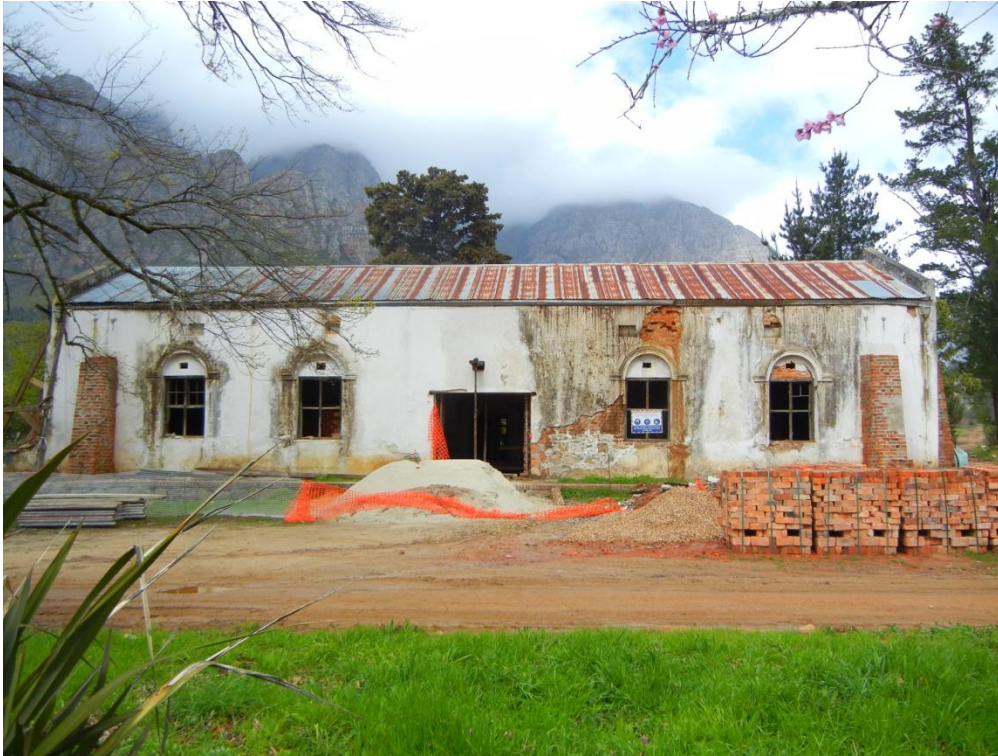
Wine Cellar Before Restoration
