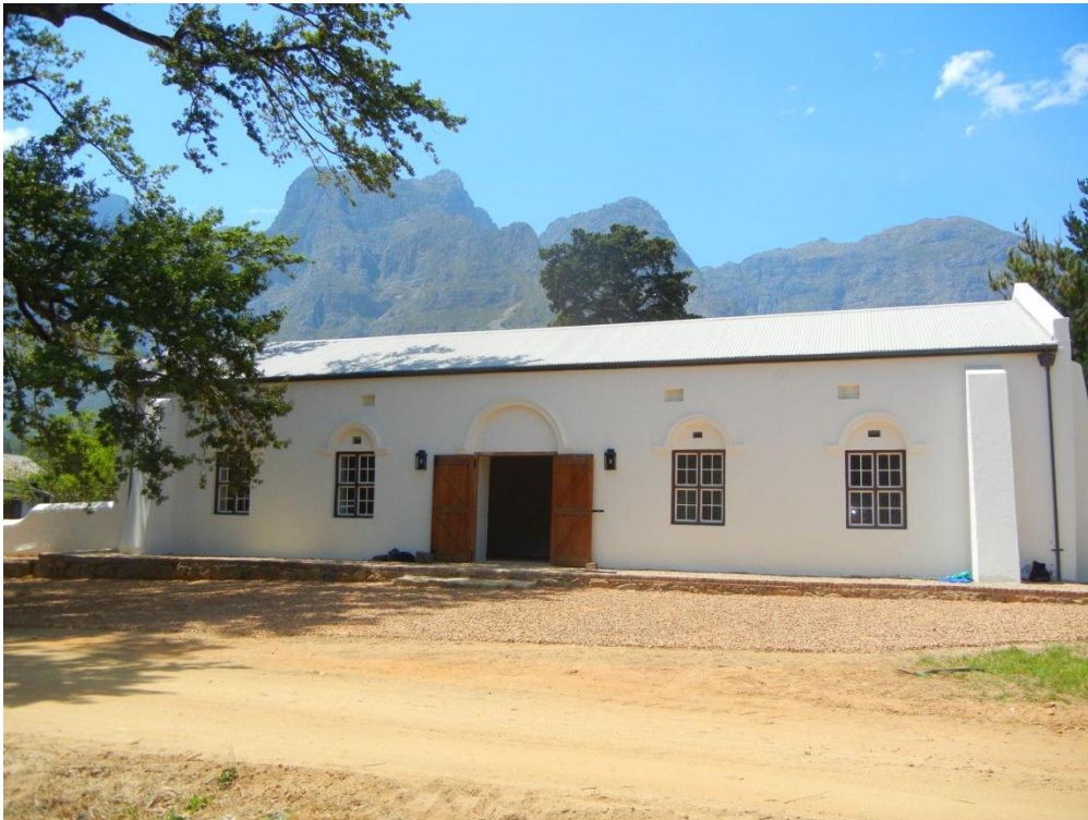
Wine Cellar after Restoration – Roof Sheetting has been replaced (First Application made to HWC in 2012)
