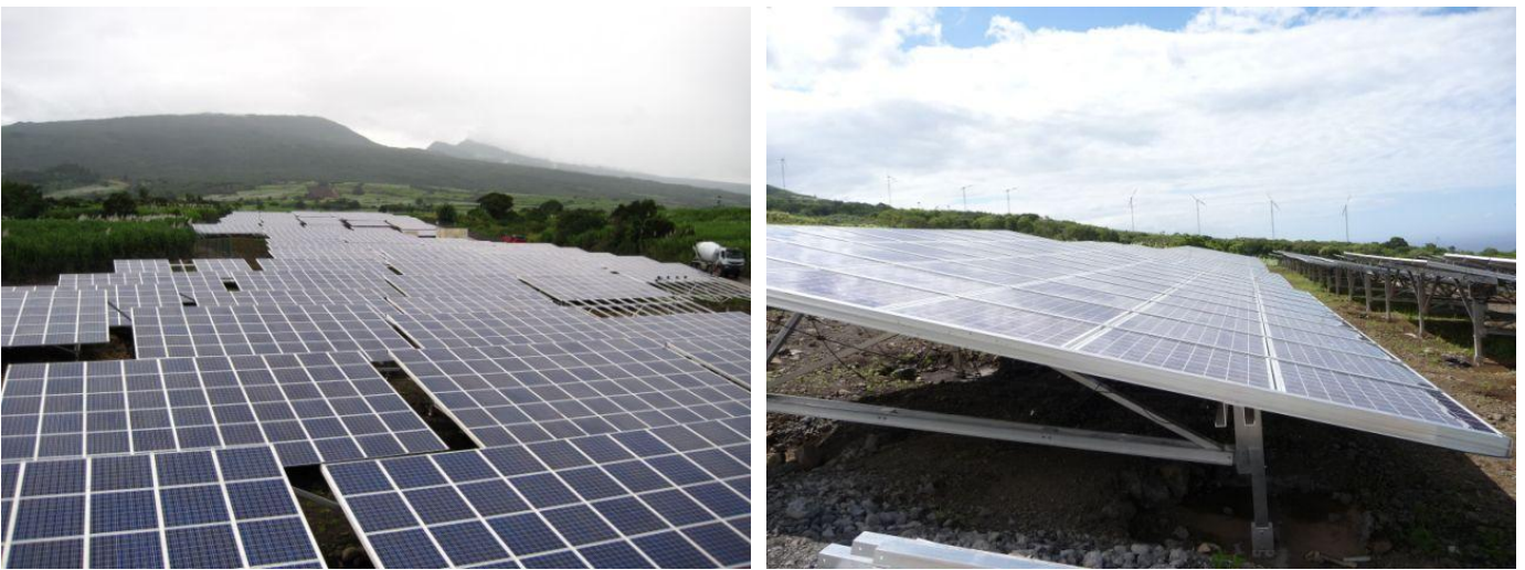
Figure 17: Fixed or rack structures
