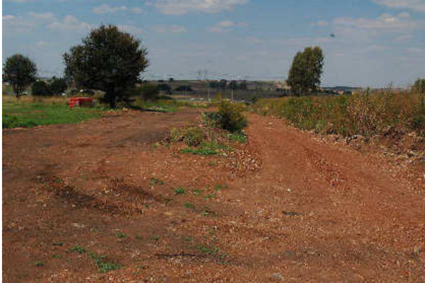
Figure 4: Road already graded east of Nellmapius Road
