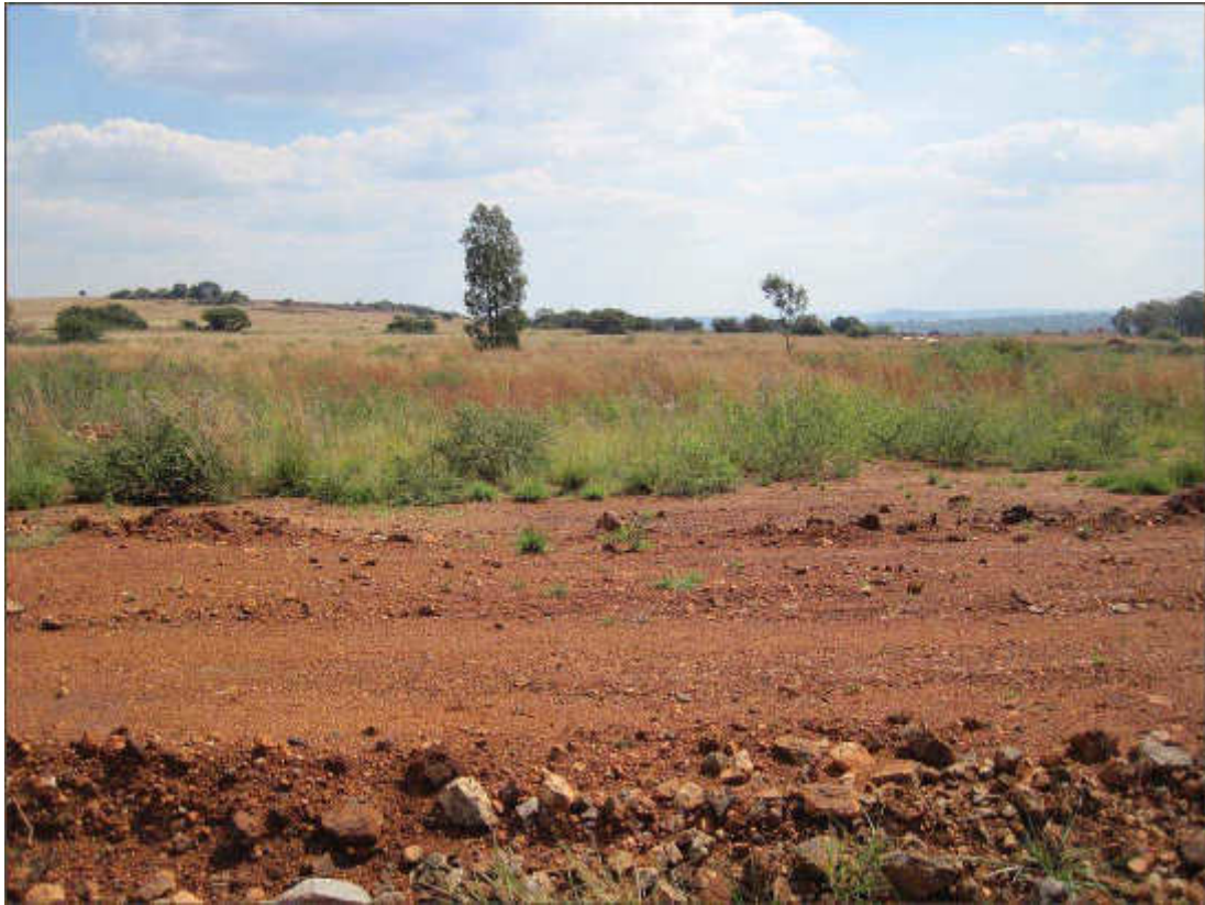
Figure 5: The point where Alternative route 2 will meet the road under construction.
