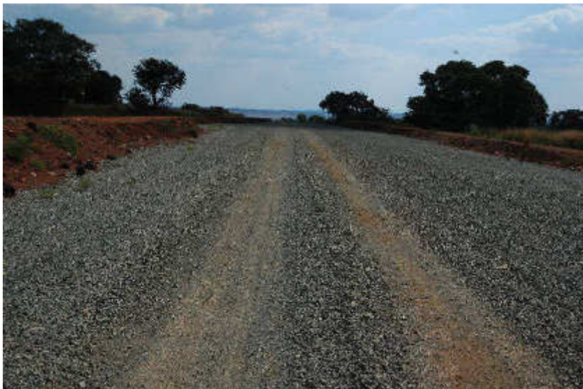
Figure 5: Road in construction
