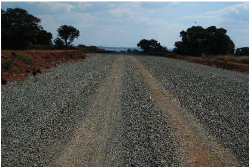
Figure 5: Road in construction
