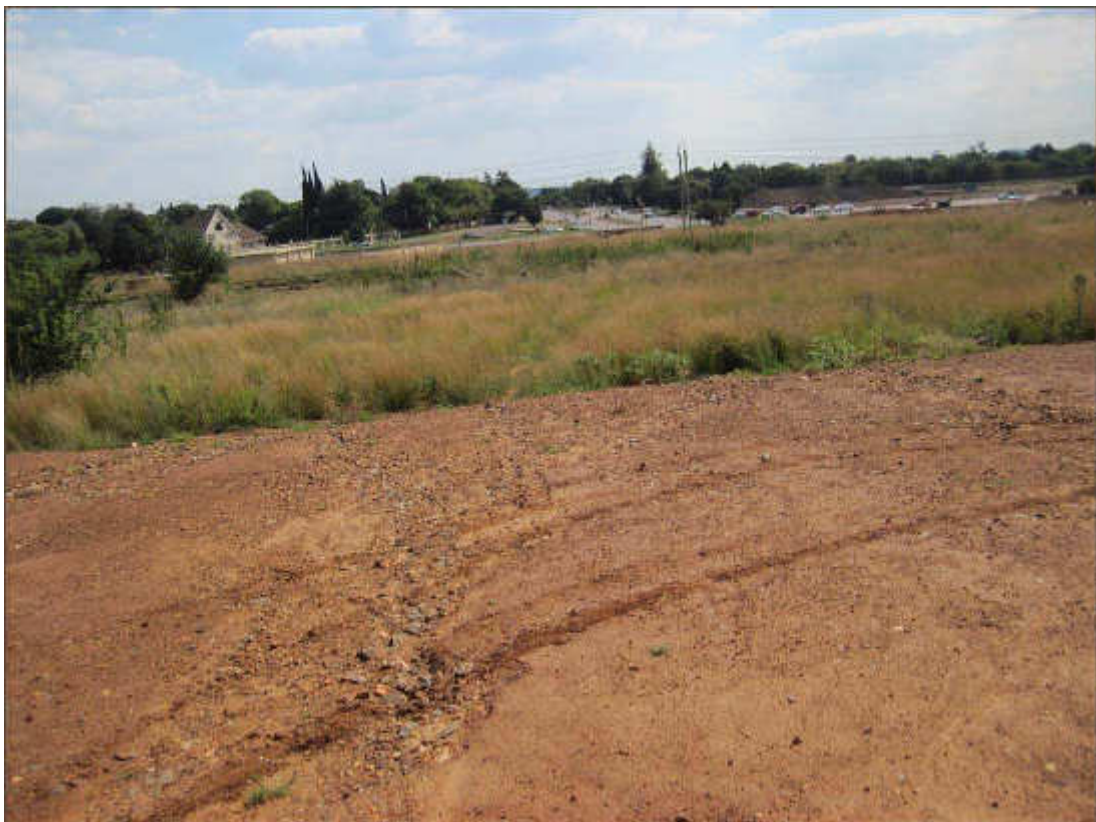
Figure 8: Where Alternative 3 will join the road under construction and cross the railway line in the foreground and link with the double lane Alexander Road visible in the distance.
