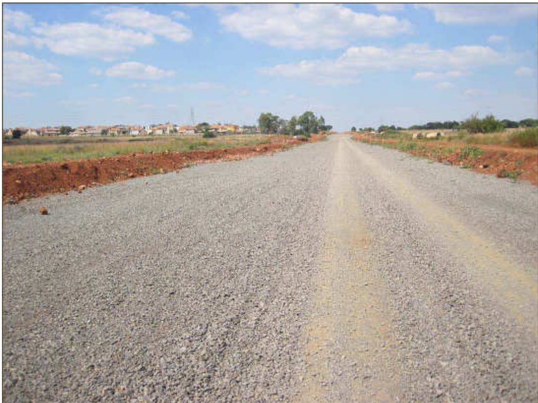
Figure 6: The point where Alternative 1 will meet the road under construction.
