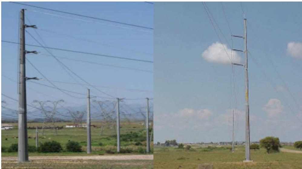
Figure 2: Typical Steel Monopole Pylon Structure
