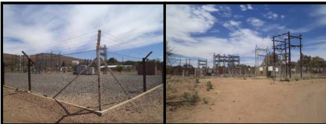
Figure 3: Existing Olifantshoek substation to be decommissioned
