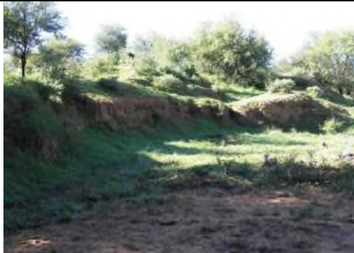
Photo 1: The deep eroded channels of the upper portion of the Olifantsloop watercourse.
