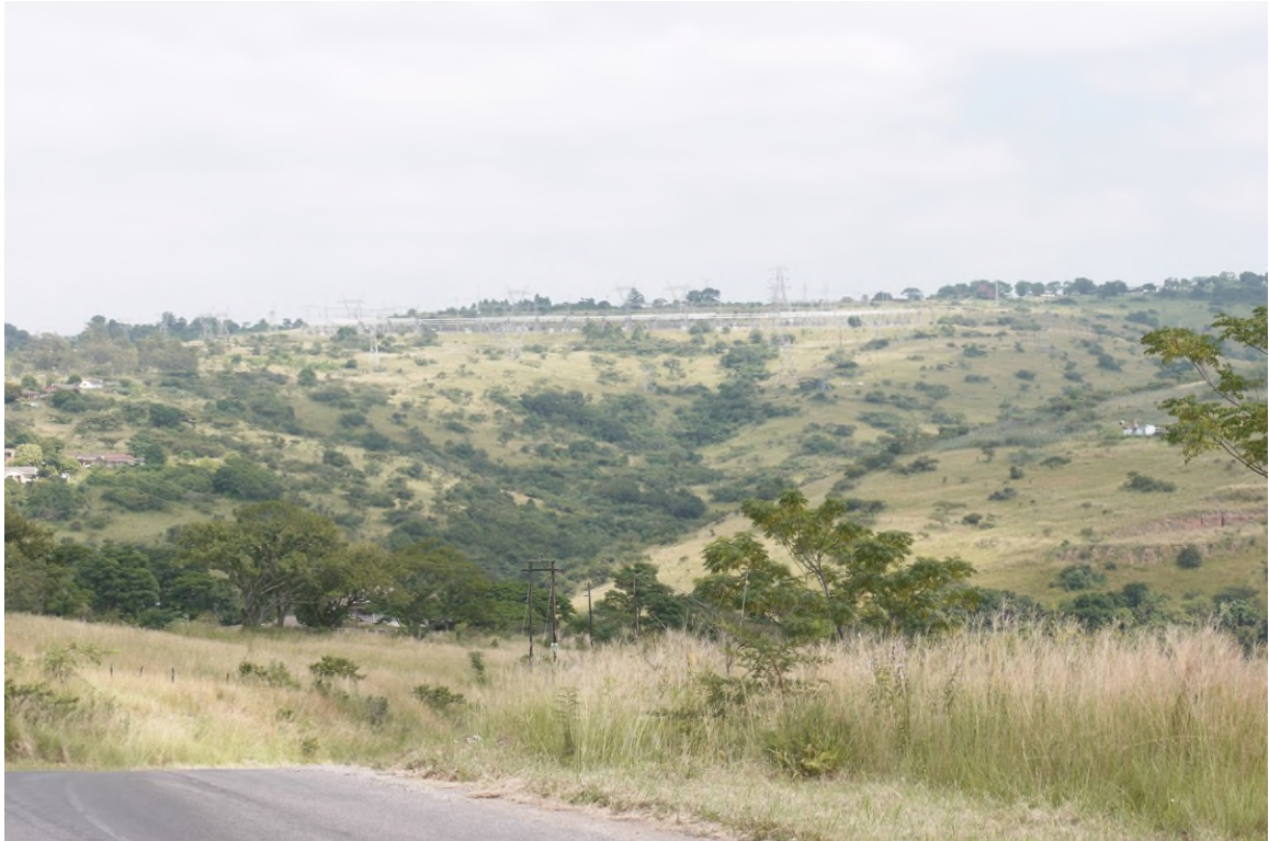
Plate 10, Distance view (1.5-2.0km) of the existing Hammersdale 400kV Substation. Note the 400kV pylons entering the site are the most obvious elements
