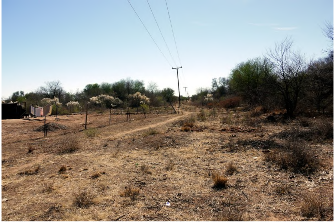
Plate 15 – VP4 looking east away from the existing substation.
