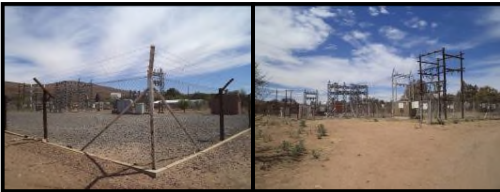
Figure 1.4: Existing Olifantshoek substation to be decommissioned
