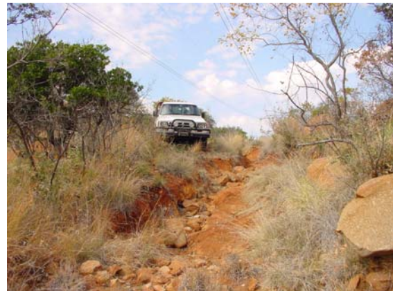
Figure 2. Examples of erosion in the servitude, which hampers access during maintenance and emergencies.
