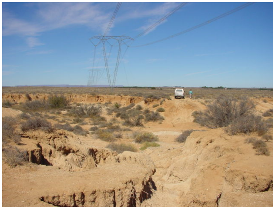
Figure 2. Examples of erosion in the servitude, which hampers access during maintenance and emergencies.
