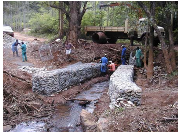
Figure 3. Extensive measures taken to prevent erosion, during the construction of access roads for a new power line. Continuous cellular mat (left) and gabions (right) are some of the measures used during the building of access roads during the construction phase of a power line. (Photos: JoseClara).
