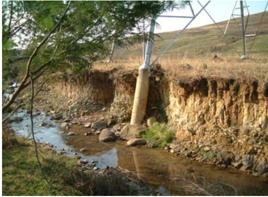
Figure 1: The photo on the left shows the foundation of a tower exposed by erosion. The photo on the right shows the extensive and costly remediation by using gabions and reno mattresses. Also note the use of good topsoil that will permit the re-establishment of vegetation around the tower (photos JorgeCorreia).
