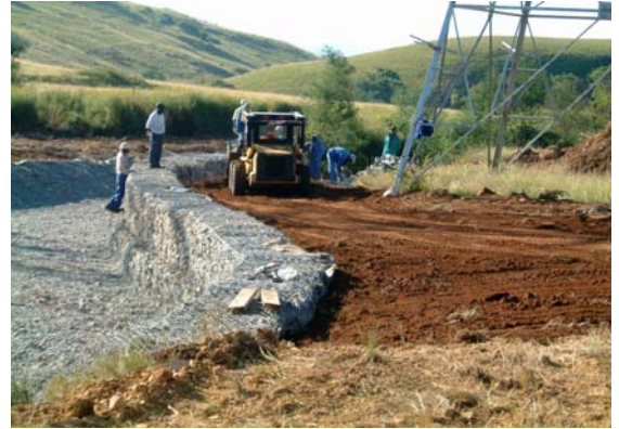
Figure 1: The photo on the left shows the foundation of a tower exposed by erosion. The photo on the right shows the extensive and costly remediation by using gabions and reno mattresses. Also note the use of good topsoil that will permit the re-establishment of vegetation around the tower (photos JorgeCorreia).
