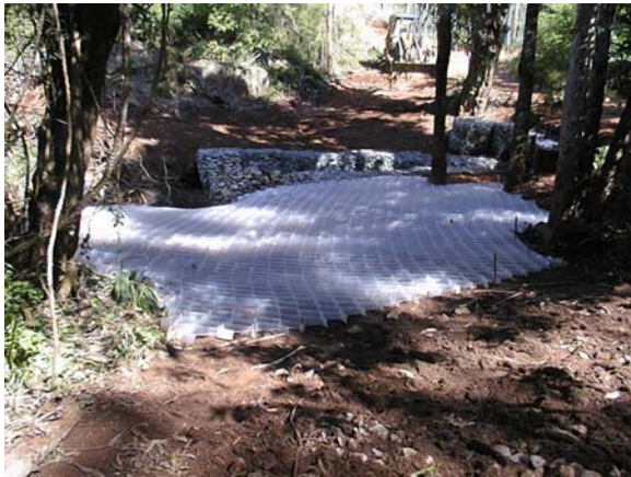
Figure 3. Extensive measures taken to prevent erosion, during the construction of access roads for a new power line. Continuous cellular mat (left) and gabions (right) are some of the measures used during the building of access roads during the construction phase of a power line. (Photos: JoseClara).
