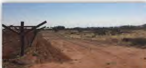
Figure 8: Scarifying of soil
