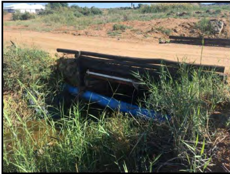
Figure 6: Stream crossing 3 – small pipelines
