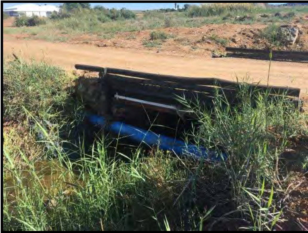
Figure 7: Stream crossing 3 – small pipelines
