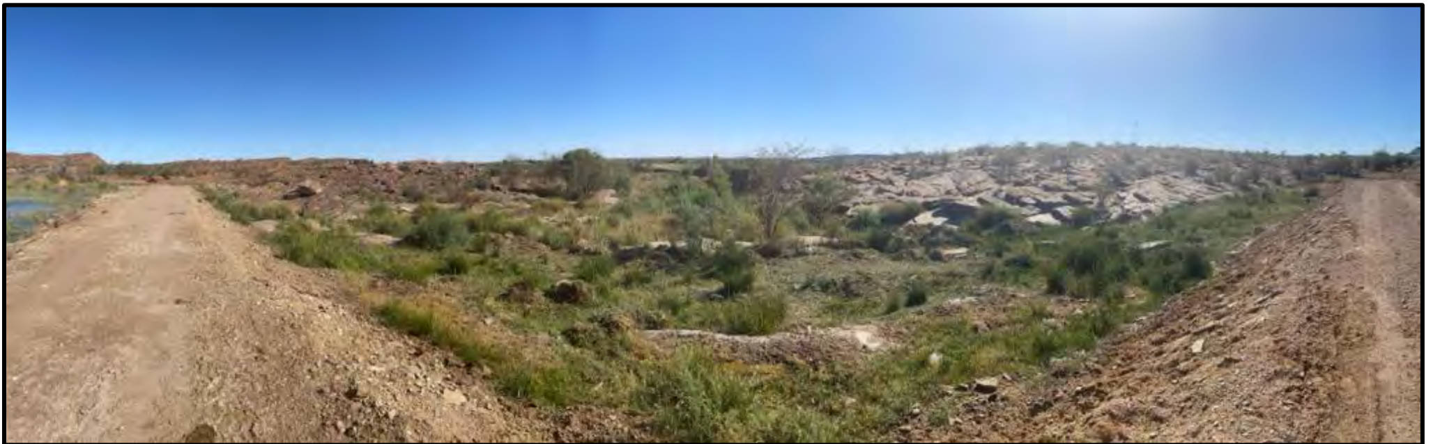
Downstream of Retention dam/wall
