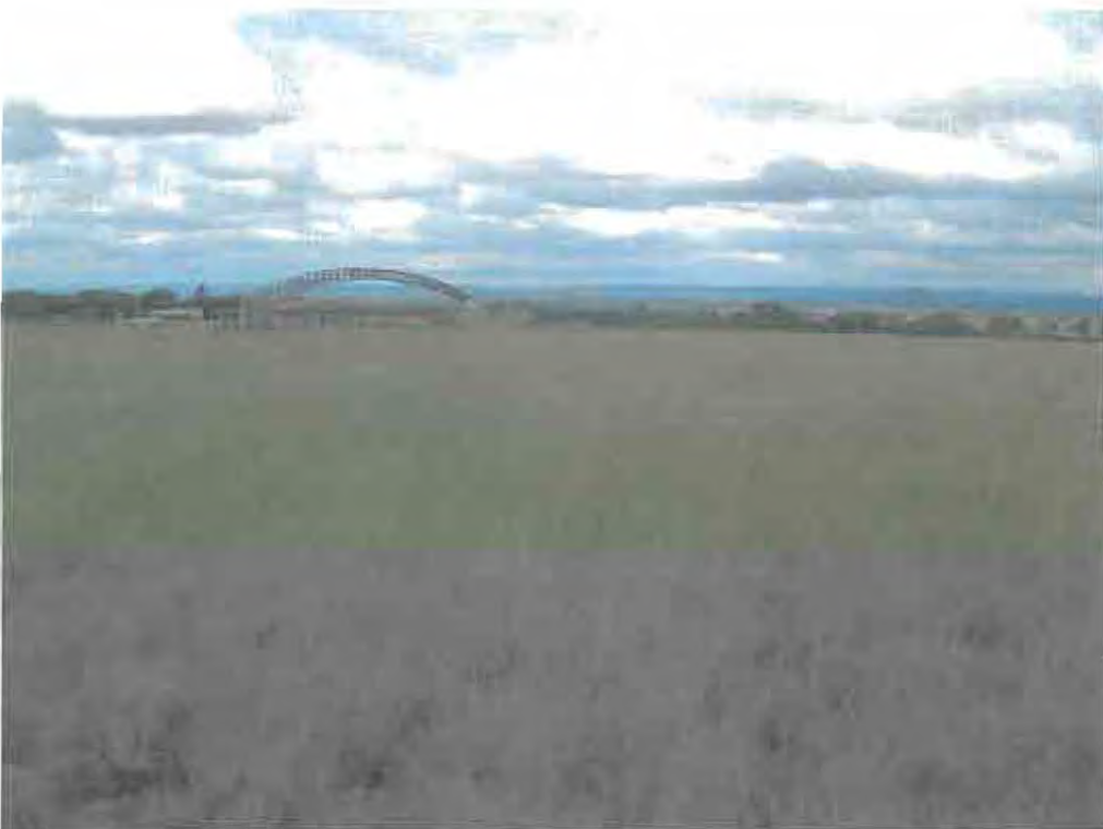
10. Half-completed church east of the site
