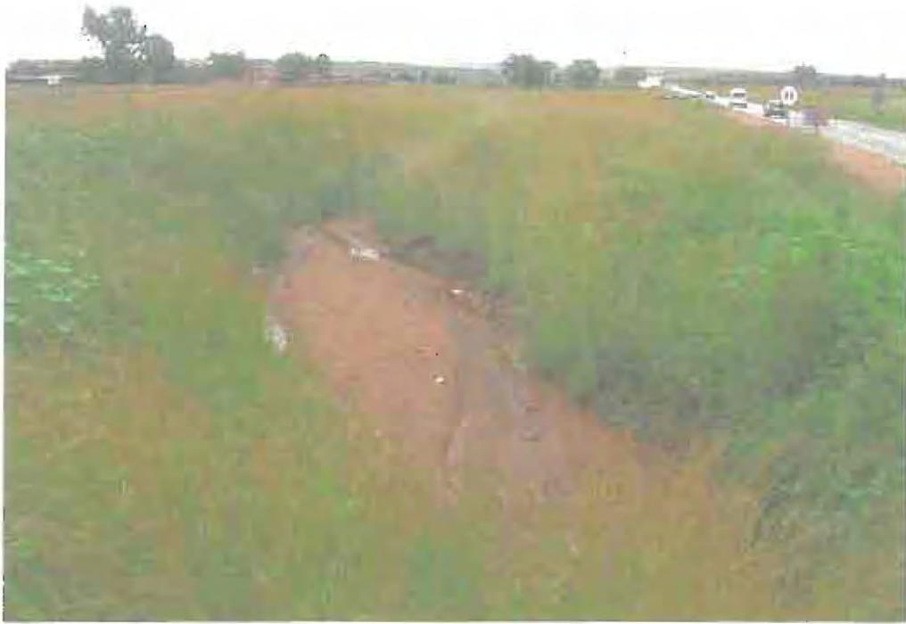
9. Drainage towards Soutpanspruit in the northeast of the site
