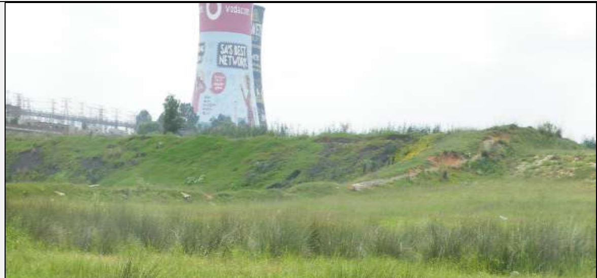
Figure 8) Bare soils on the dam wall
