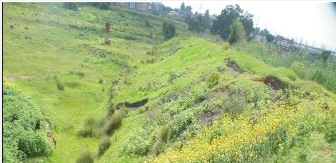
Figure 9: Eroded dam wall
