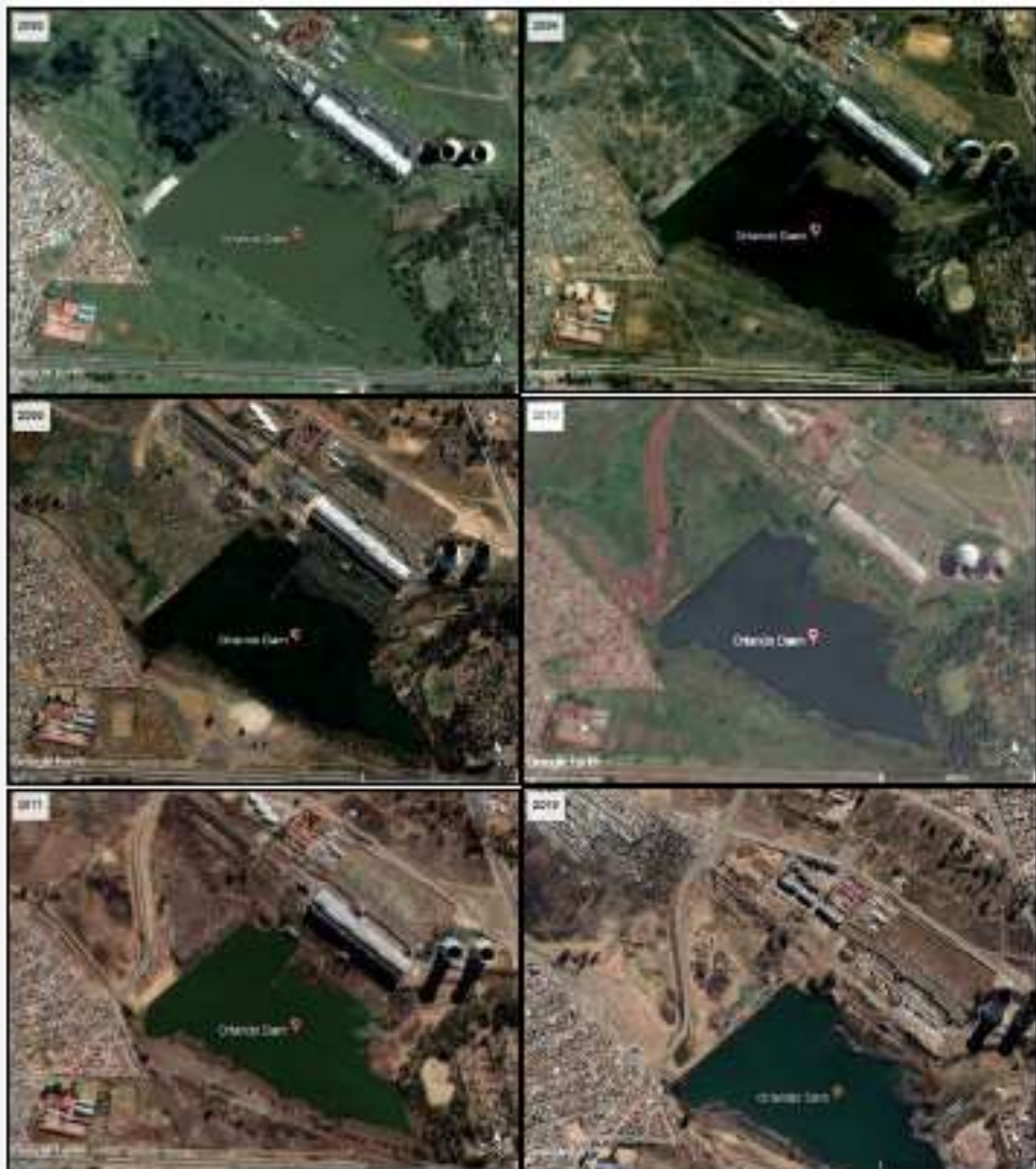
Figure 1: Google Earth aerial imagery of the dam and surrounding vegetation from 2000, 2004, 2006, 2010, 2011 and 2019 show the continuous soil disturbances around the dam over time
