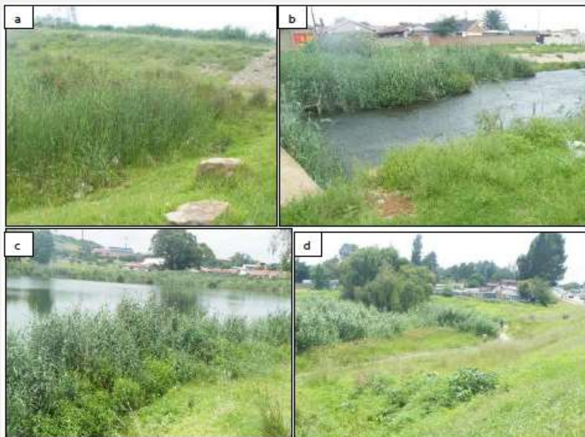
Figure 14: a) P. australis in the pond underneath the dam overflow north of the dam wall, b) P. australis in the spillway, c) around the edge of the dam and d) at the inflow of the Diepkloofspruit at Chris Hani Road.
