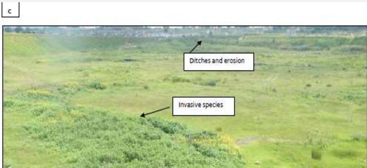
Figure 7c: Vegetation north of the dam wall- ditches and invasive plant species were common.
