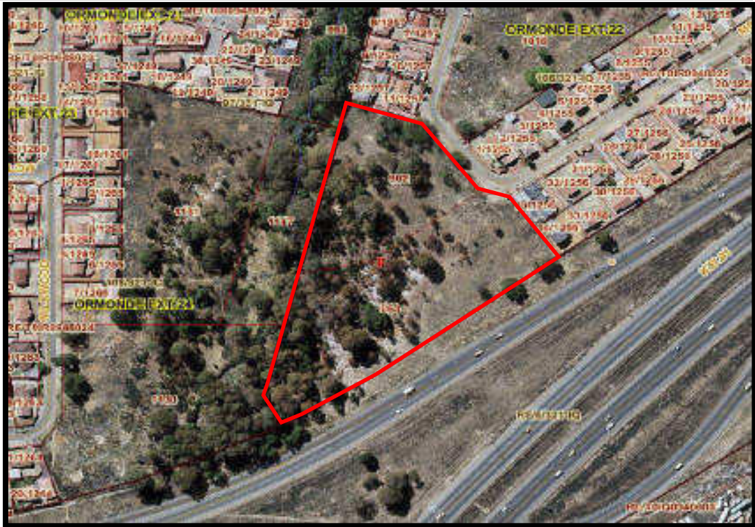
Figure 1: Aerial view of the property
