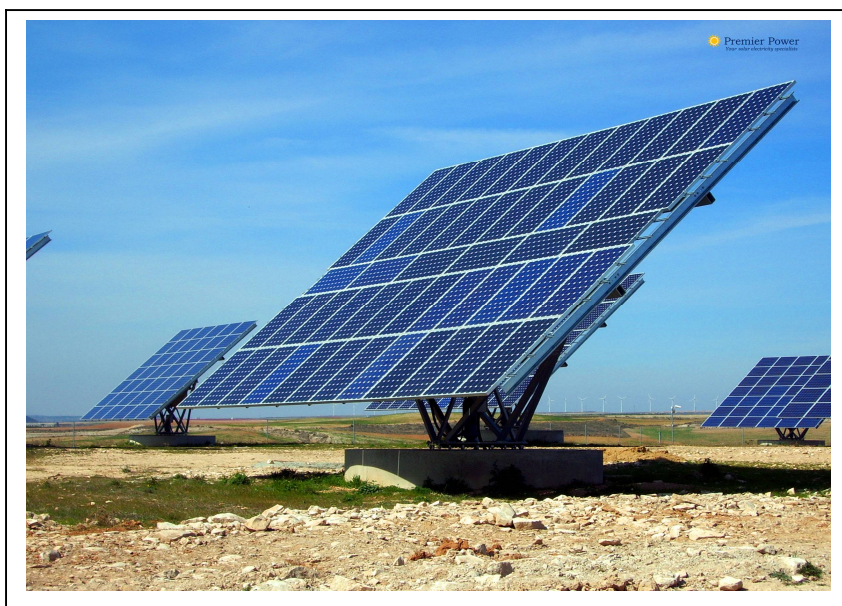
Figure 2.3: The support structures elevate the panels and allow for dual axis tracking of the sun for increased efficiency (Source: Gigaom)
