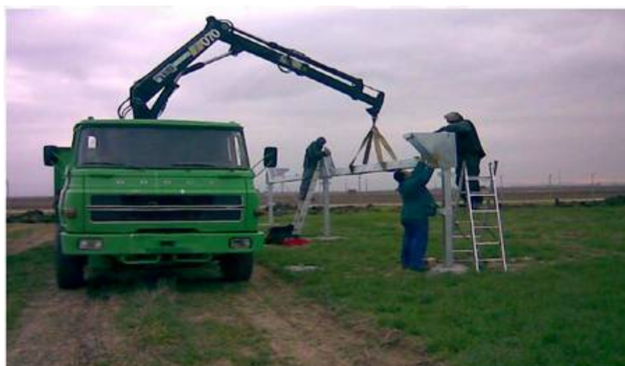
Figure 2.4 Mounting of the frame for the PV panels (Courtesy of Igeam, 2011)
