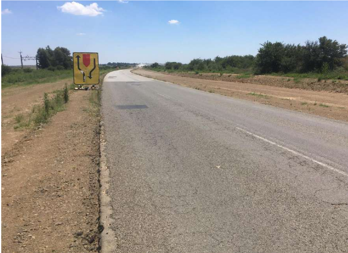
Figure 3-9: Construction on R76
