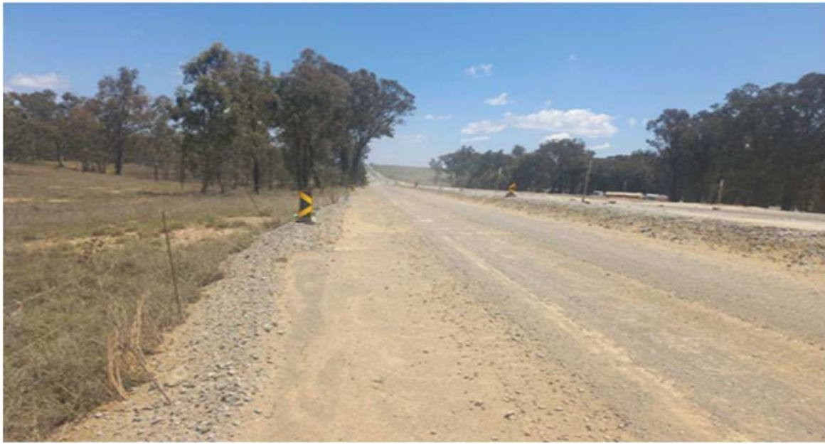
Roadworks along the R76
