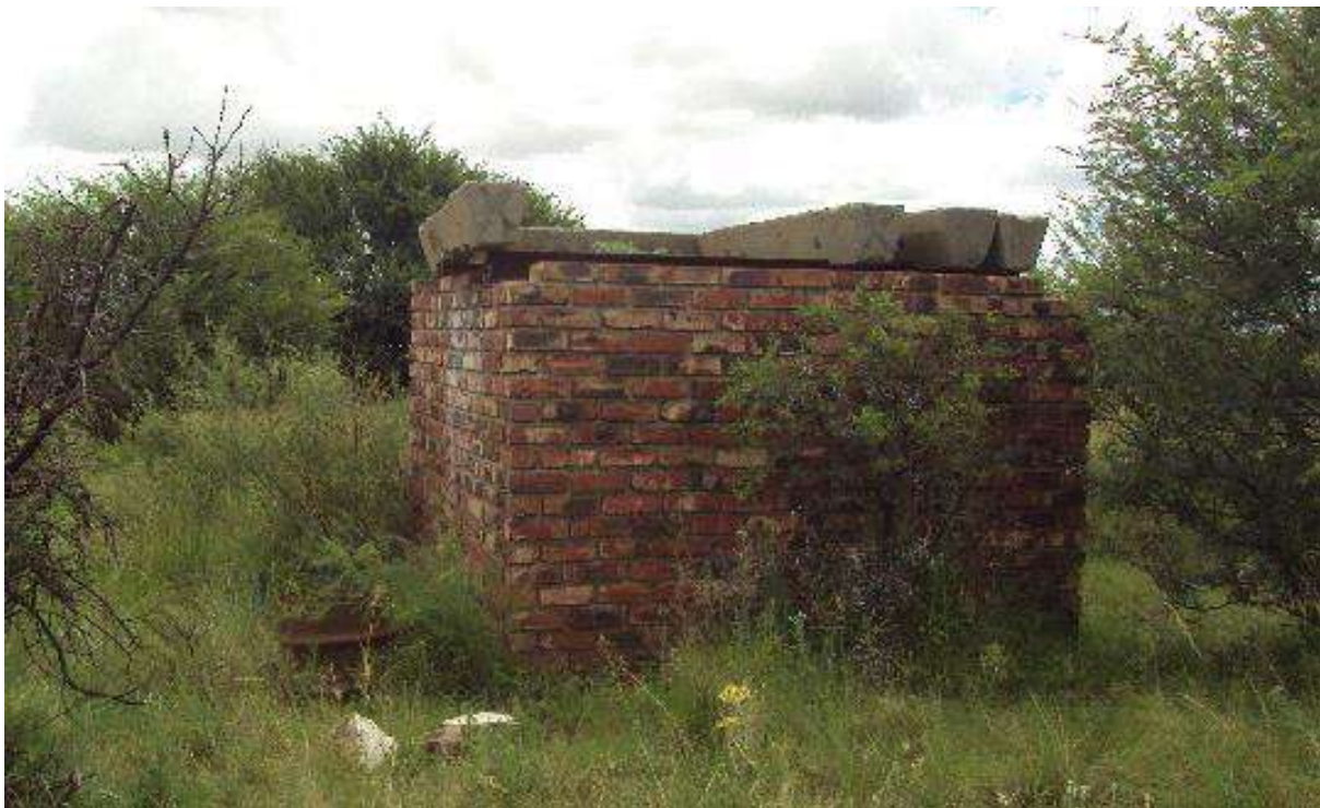
Figure 15: View of support structure for water tank (Site Os2-01)
