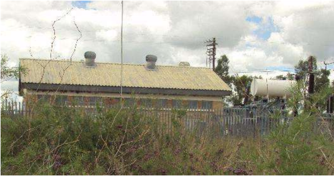
Figure 18: View of western elevation of the substation building, Os2-03
