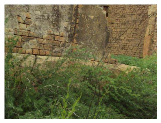
Figure 51: View of the farmhouse construction materials; showing sandstone foundation, mud bricks and commercial bricks
