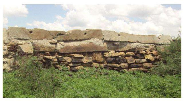
Figure 55: View of kraal wall, showing past repair work
