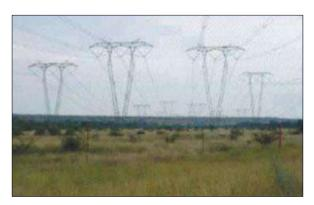
Figure 8: 400kV guyed V-Tower Structures
