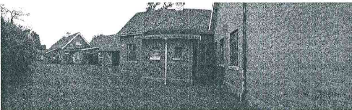
Back Elevation of OT Building
