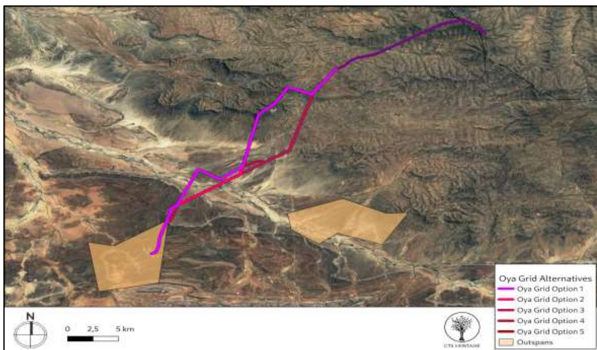
Figure 43: The proposed alignment alternatives for the Oya OHL grid connection and substation sites relative to known outspans in the area
