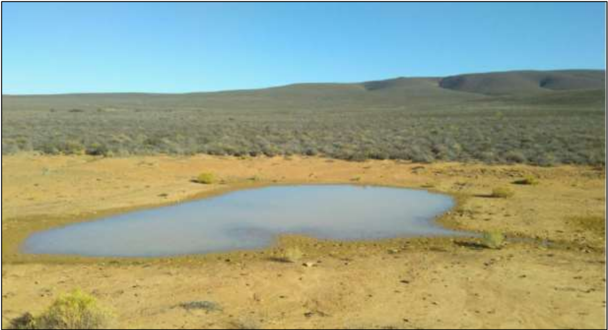
Figure 33: An earth dam in the study area
