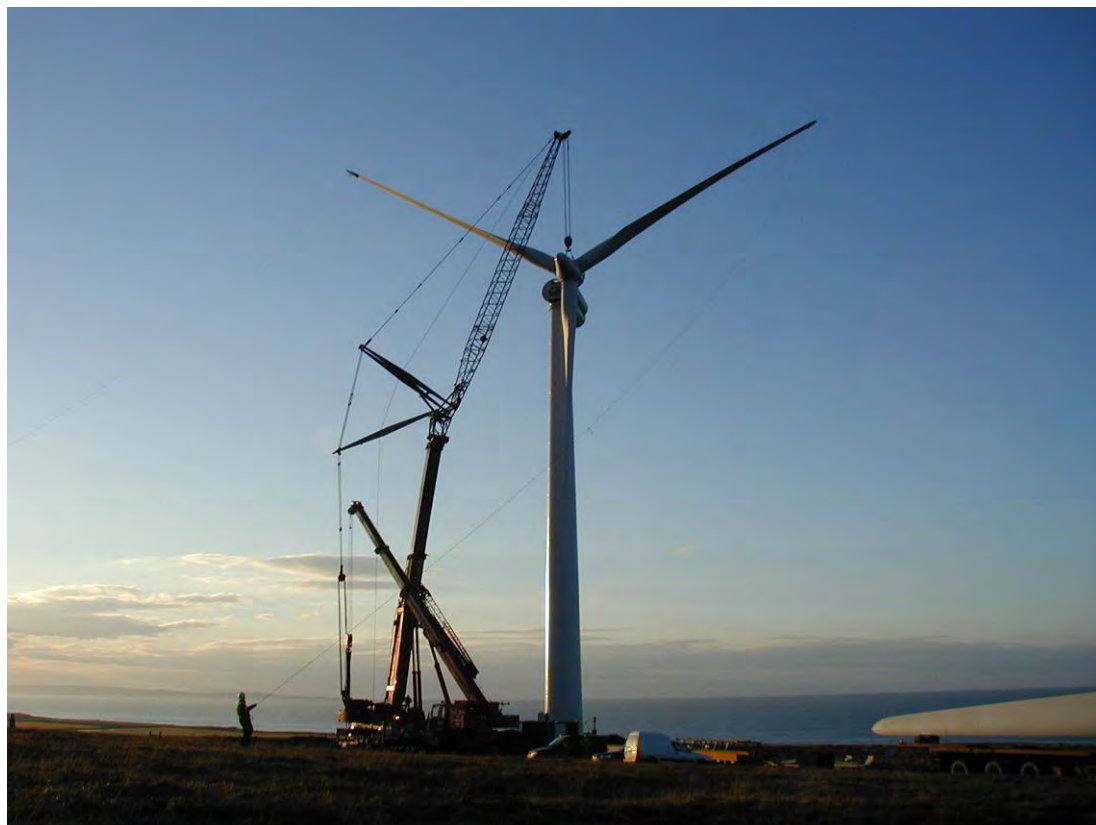
Figure 3.10: Lifting of rotor blades during erection of turbine
