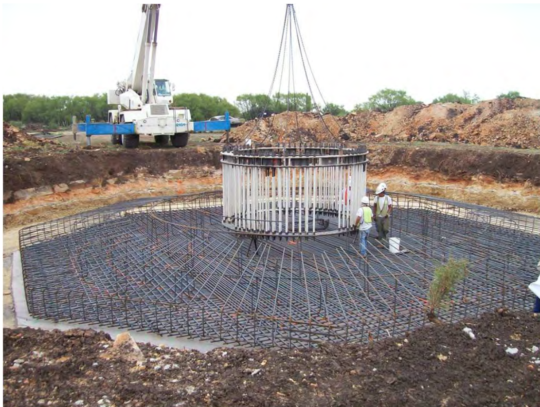
Figure 3.6: Construction of turbine foundation
