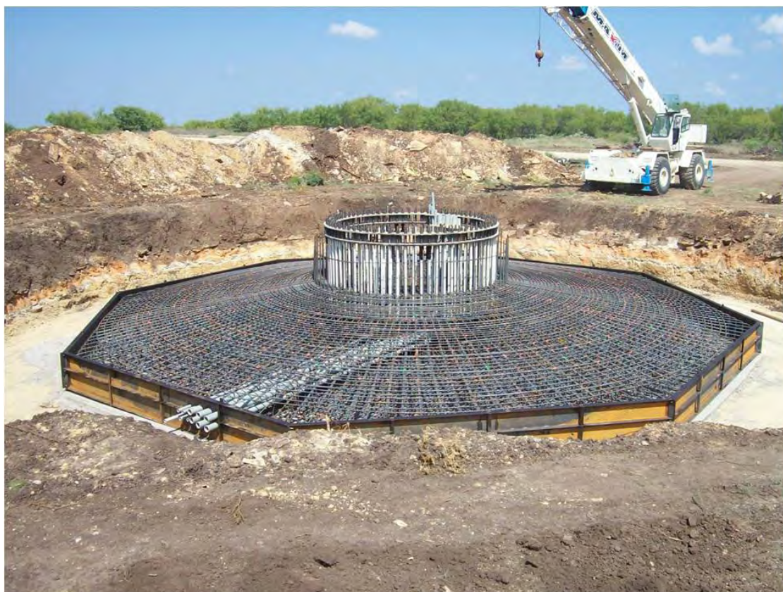
Figure 3.7: Construction of turbine foundation
