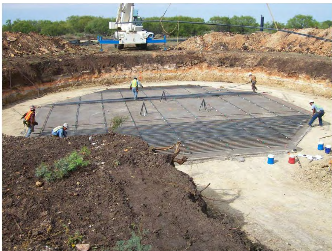
Figure 3.5: Construction of turbine foundation
