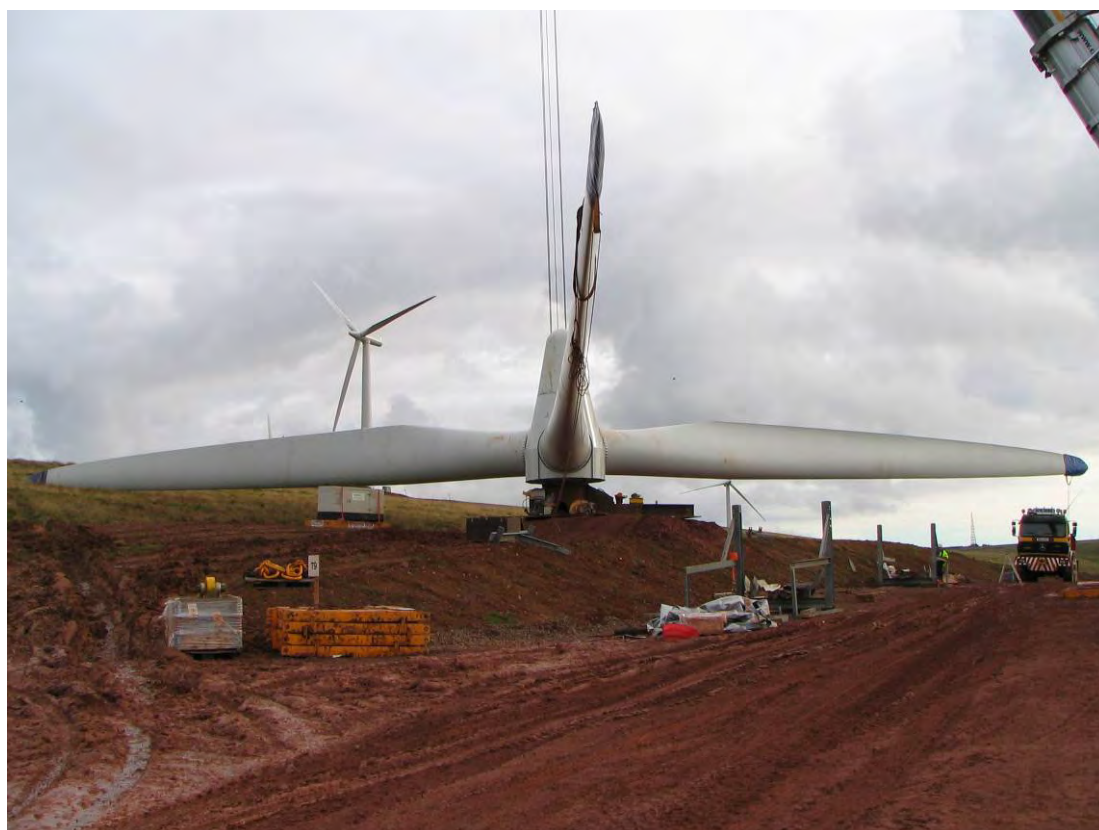
Figure 3.9: Lifting of rotor blades during erection of turbine
