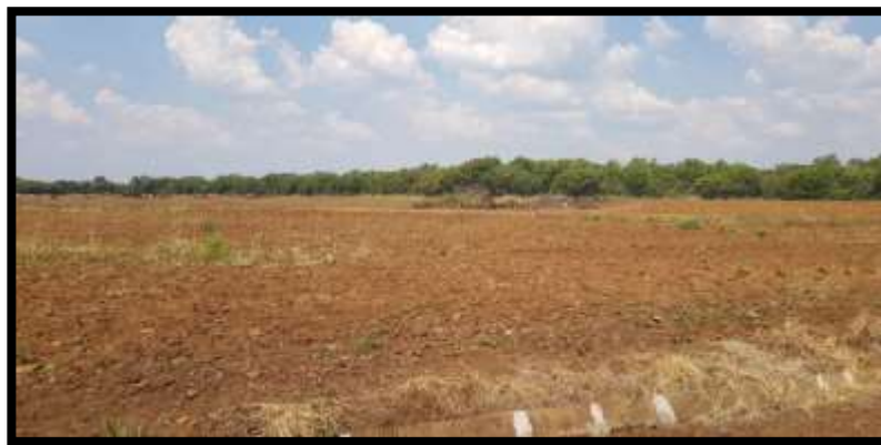
Photo 4: Vegetation cleared in order to erect Chicken Broiler Houses.
