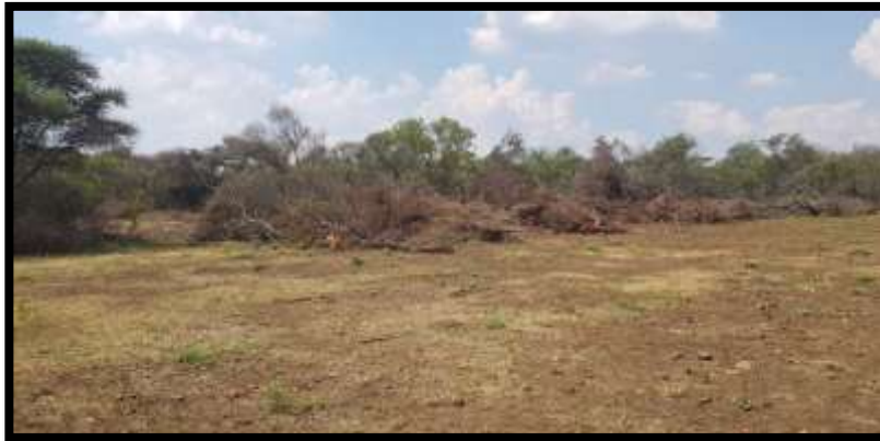
Photo 3: Vegetation cleared in order to erect Chicken Broiler Houses.
