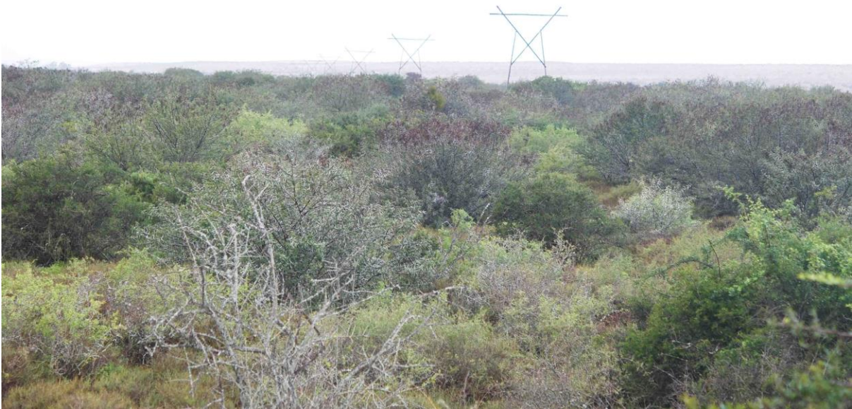
Figure 35: View eastward along pylon route from point 27 (Fig.1). Recent alluvium underlies the route in the foreground.
