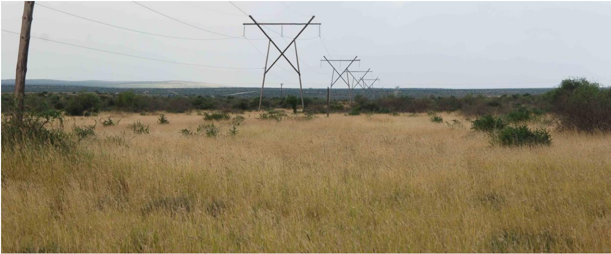
Figure 36: View looking eastwards, along pylon route across plain of weathered Kirkwood Formation, from point 28.
