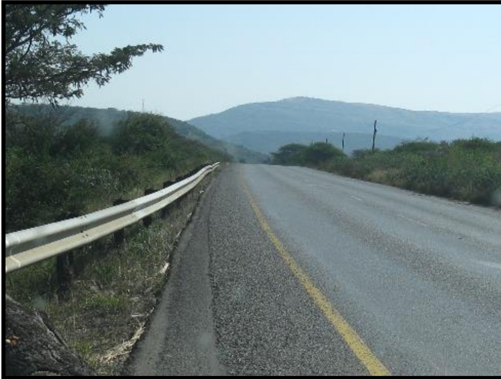
Figure 5. The western section of the P230.
