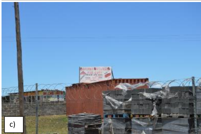
Photograph 2: a) Caltex Service Station situated along P483; b) Cashbuild store and Dry cleaning services situated along P483; c) Building blocks supply store situated along P483
