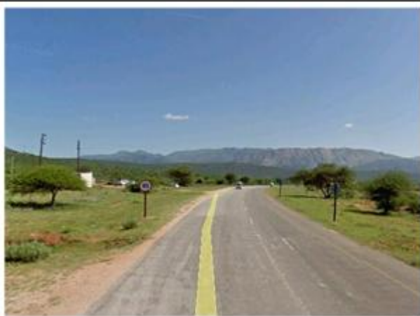
Photo 3: Paved road to Mafefe which bisects the proposed project area.
