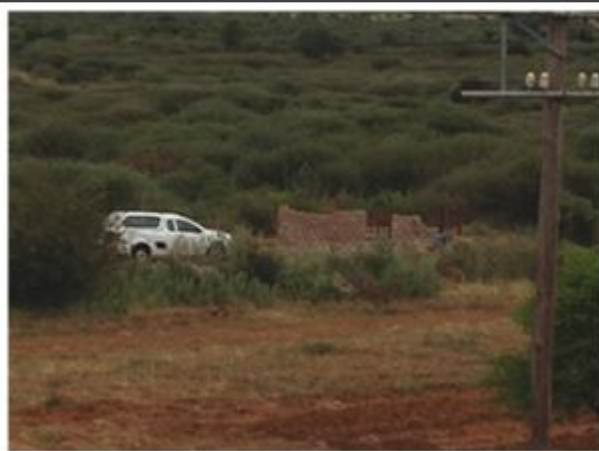
Photo 4: Small informal building being constructed within the proposed project area.
