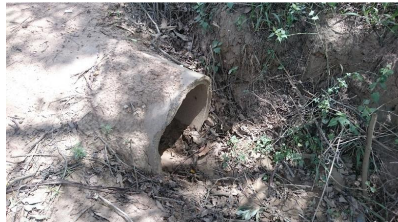
Photograph 8: Shows a stormwater surrounded by sediment which will either build up overtime and block the pipe or in heavy rainfall, be washed down the steep banks and cause erosion.
