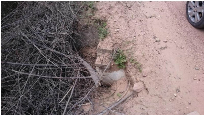
Photograph 7: Shows one of the culvers along road P75-2, which is seen to be blocked and eroded.
