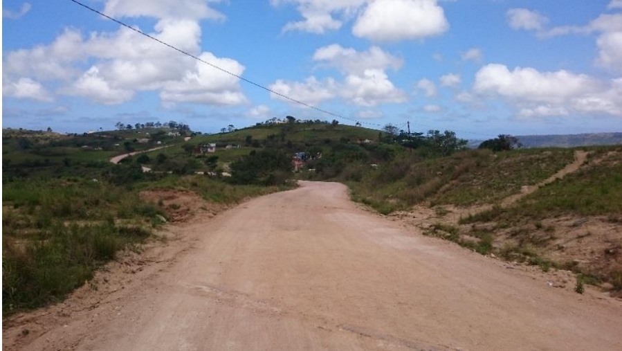
Photograph 1: Shows the existing condition of road P75-2
