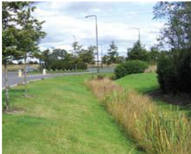
Example of a swale alongside a road.
