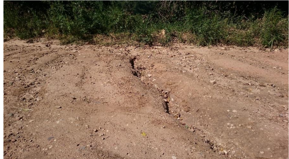
Photograph 4: Shows the existing condition of road P75-2 and the erosion that is currently occurring. This clearly shows rutting of the road.
