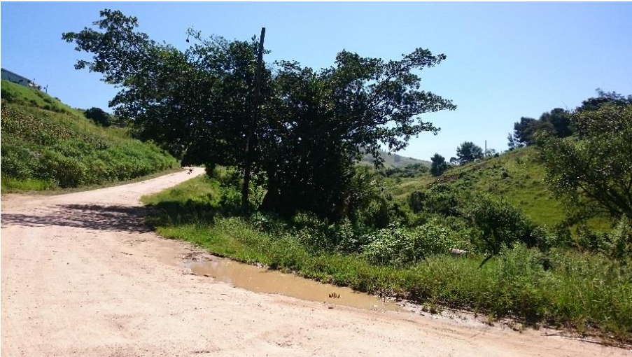
Photograph 3: Shows the existing condition of road P75-2. Note, no storm water management system has been provided, resulting in pooling of water.
