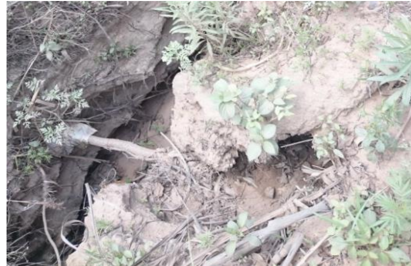
Photograph 6: Shows erosion found alongside road P75-2 due to the lack of storm water control.
