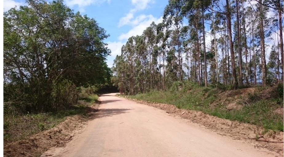
Photograph 2: Shows the existing condition of road P75-2. Note, no storm water management system has been provided.
