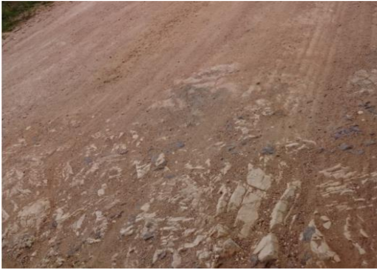
Photograph 5: Shows the condition of the road and erosion exposing rock.
