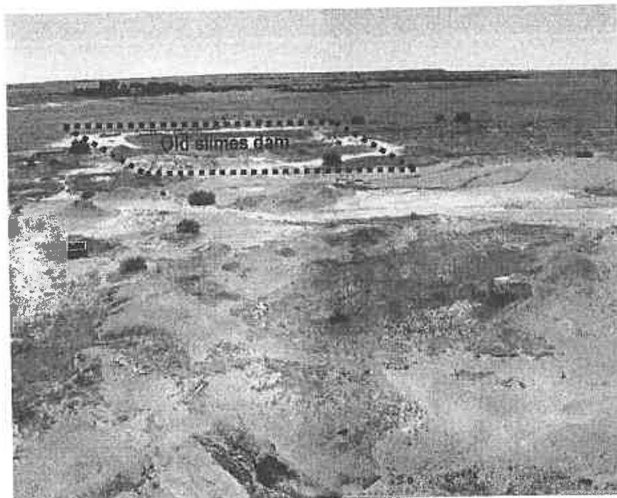
Figure 3: Existing slimes dam
