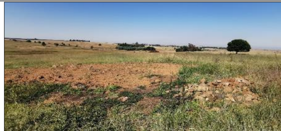
General view of the site DFN006, identified during the phase two fieldwork, showing the ground clearing activities in the surrounding area.
