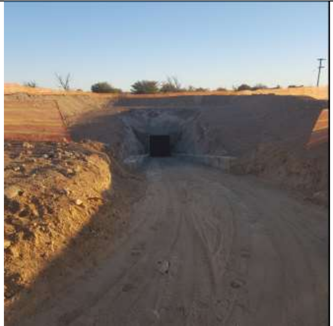
Decline Ramp Portal
