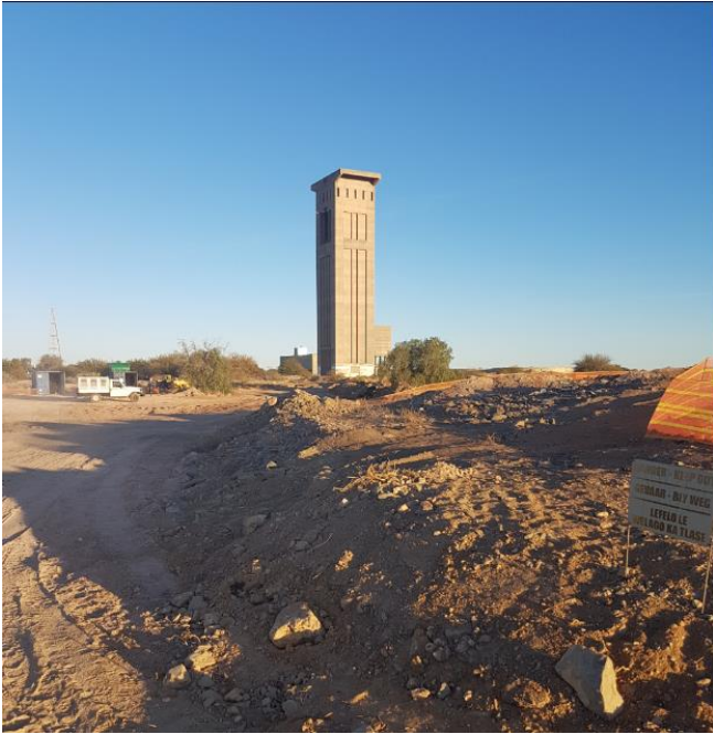
Hutchings Shaft Column
