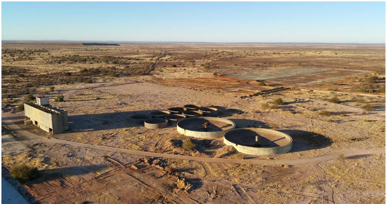
Other historical mining infrastructure remaining onsite includes the Crusher Bins, (left), Flotation Dams (middle foreground) and Concrete Drying Beds (right background)
