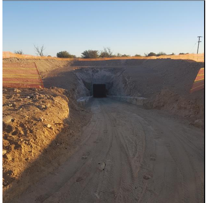
Decline Ramp Portal
